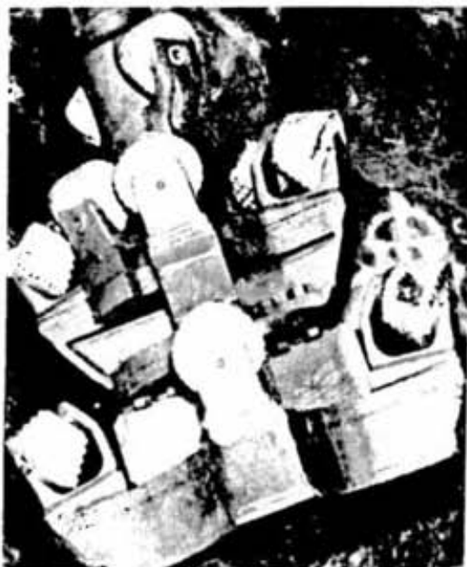
This old-style five-foot reaming head was called a "Christmas tree" because of its shape and its 12 cutters which resembled ornaments. Compare with the flat seven-foot head on page 9.
