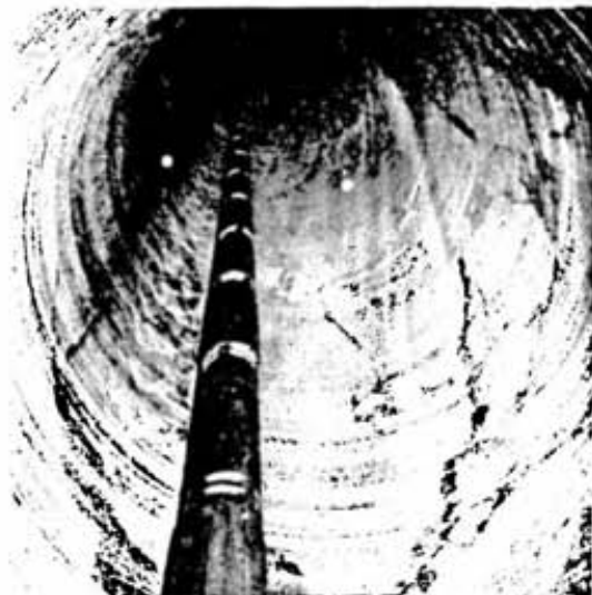
Looking up the partially completed ore pass, the shaft is the 10-inch drill rod to which the reaming head is attached. The smooth-walled circular hole is preferred when the raise is to be used for ventilation. Air resistance is much lower than in a conventionally drilled and blasted rectangular hole.
