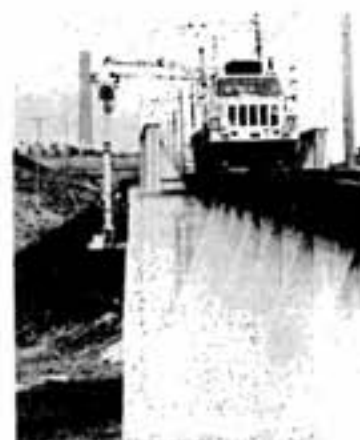
The hydraulic arm slowly extends down the side of the bridge where Inco engineer Bob Catto can begin his close-up examination of the structure's integrity and general state of repair.
