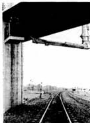
By the end of the mechanical arm's extension, it has brought the inspection crew 270 degrees around the bridge allowing for a thorough inspection.
