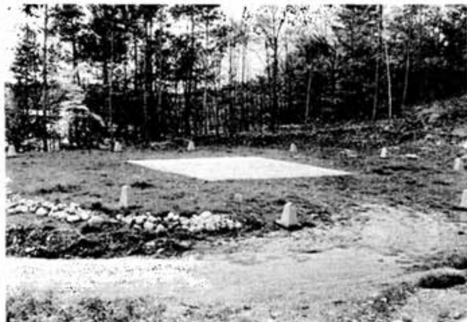
The reflective cones surrounding the heliport site allow the air ambulance to land day or night.
