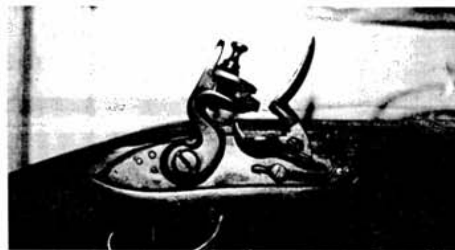
This carefully crafted flintlock was filed and created entirely by hand.
