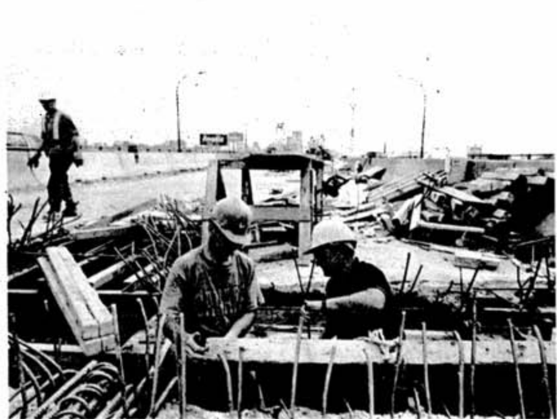
Workers struggle with corroding rebar on the Gardiner Expressway in Toronto. Decaying infrastructure represents a potential large opportunity for nickel stainless steel.
