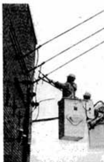
Linemen John Cowx and Cam Duncan cut the live 6,900 volt feed to #1 substation.
