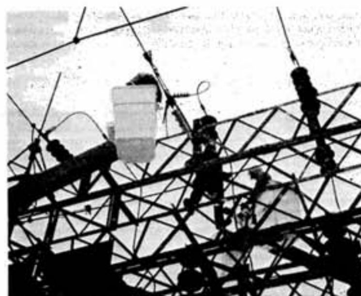
Power department linemen change substation insulators at the Copper Cliff Nickel Refinery.
