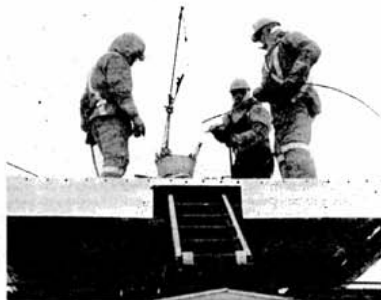
Linemen Kerry Burden, Mark Paaanen and Gaetan Denis prepare to install new trolley wire on the Frood main line.
