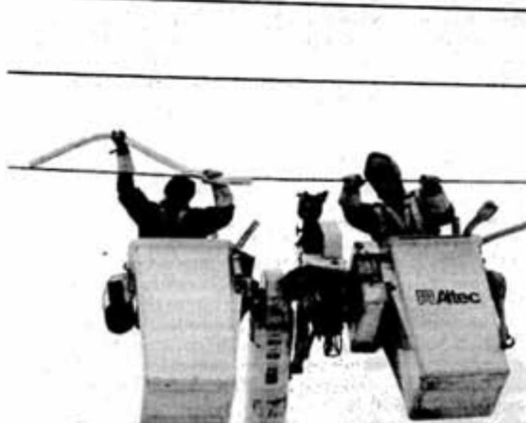
Linemen John Cowx and Cam Duncan install rubber insulating cover-up to protect themselves from the live 6,900 volt phases. They then install an in-line switch on the live 6,900 volt general circuit.
