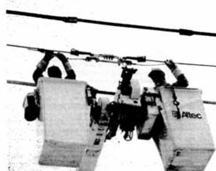
Linemen John Cowx and Cam Duncan install rubber insulating cover-up to protect themselves from the live 6,900 volt phases. They then install an in-line switch on the live 6,900 volt general circuit.
