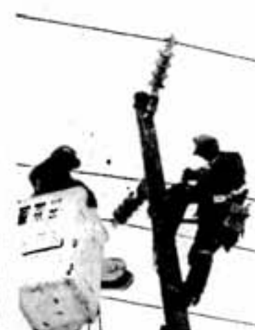
Linemen Karl Bubalo (on the pole) and Marty Makela change insulators on the Nickel Refinery power line.
