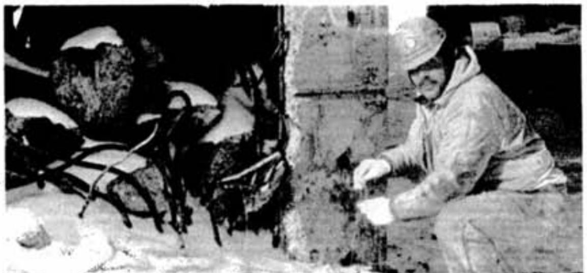
Al Corby of Engineered Demolition performs a final check on the blasting wire connections to ensure everything is set for the blast.
