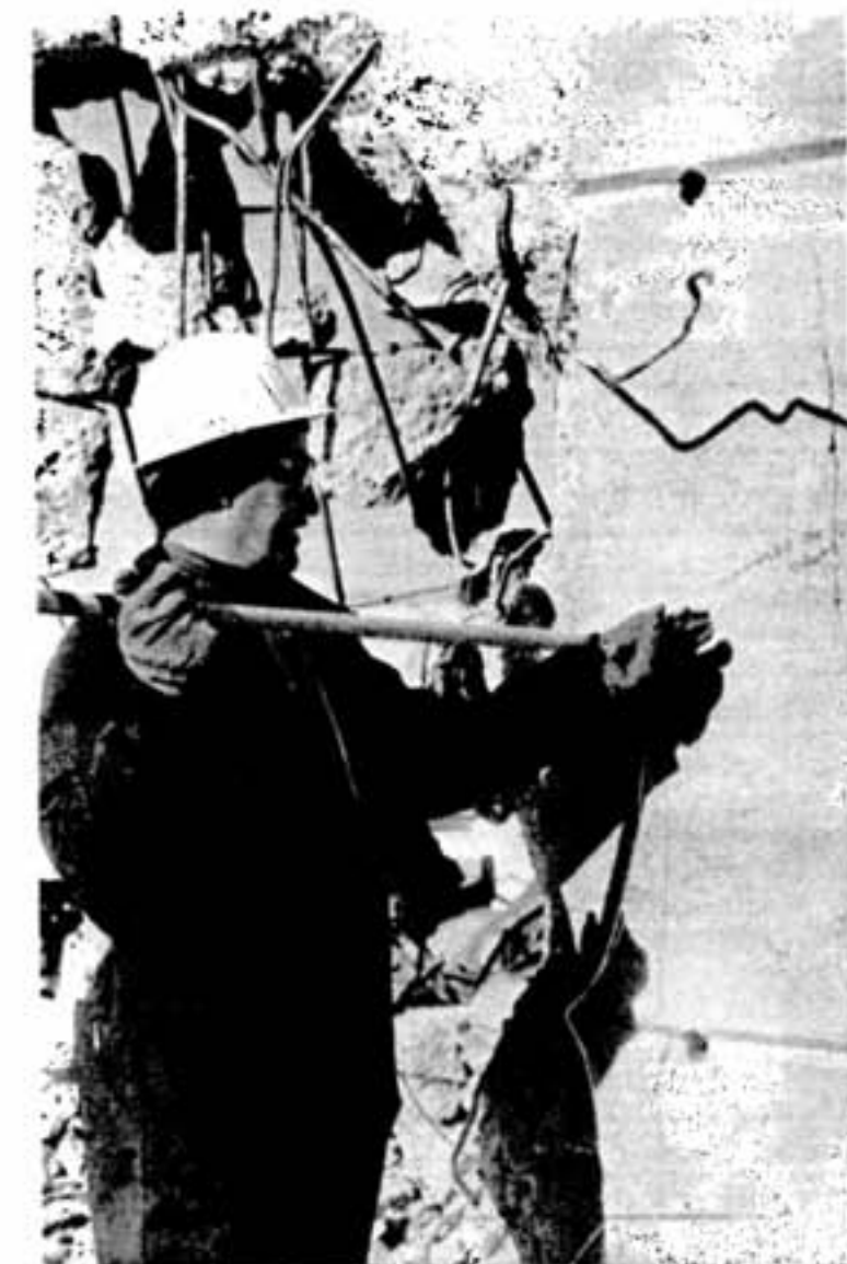
Mark Patrakka of Corona Inc. in Lively loads the explosives that would help topple the large concrete headframe.
