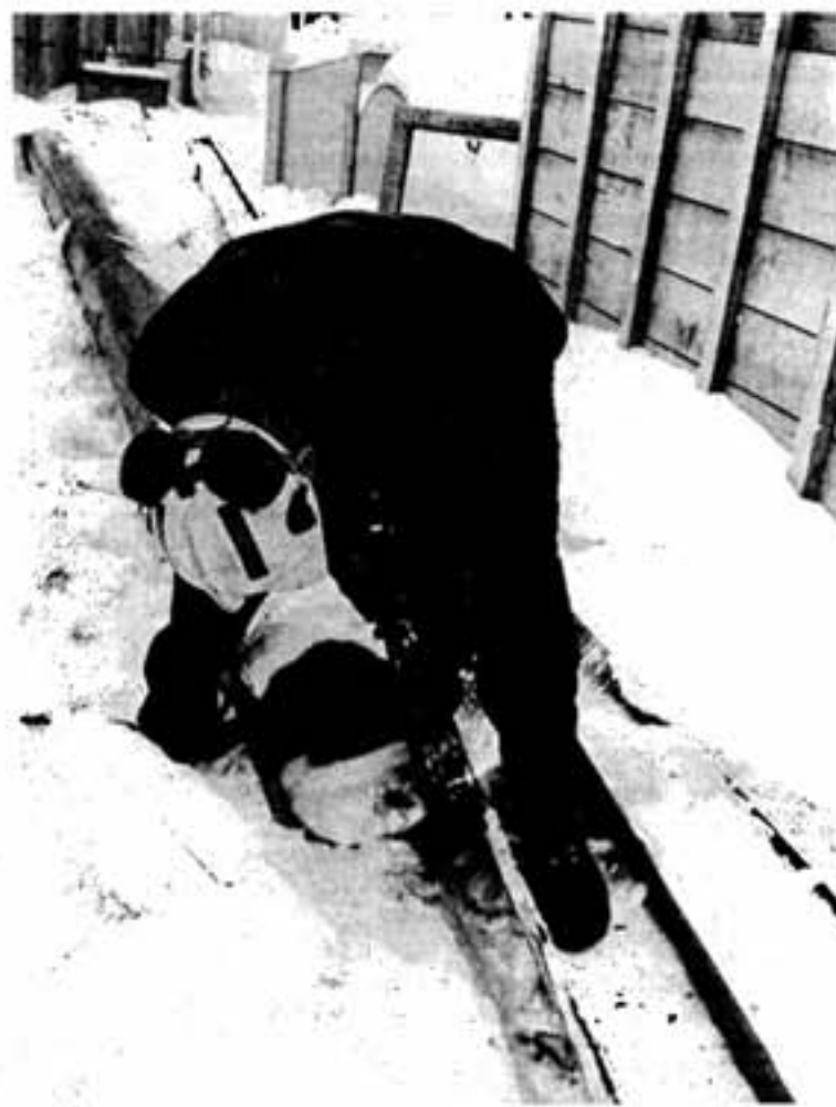
Industrial mechanic Yvon Delay of the Power department cuts an H-beam with a blowtorch. Yvon said talking over a job with a fellow employee is a good first step to working safely.
