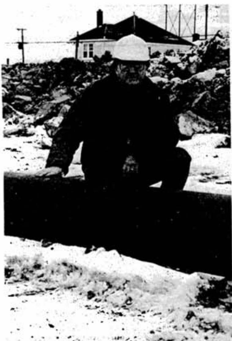
This new line will allow sludge from the Copper Cliff Waste Water Treatment Plant to be pumped directly to Booster Station, enabling the shutdown of four pumps in the process, said Tom McDonald. Previously, the sludge was routed through Copper Cliff Mill before reaching Booster Station.
