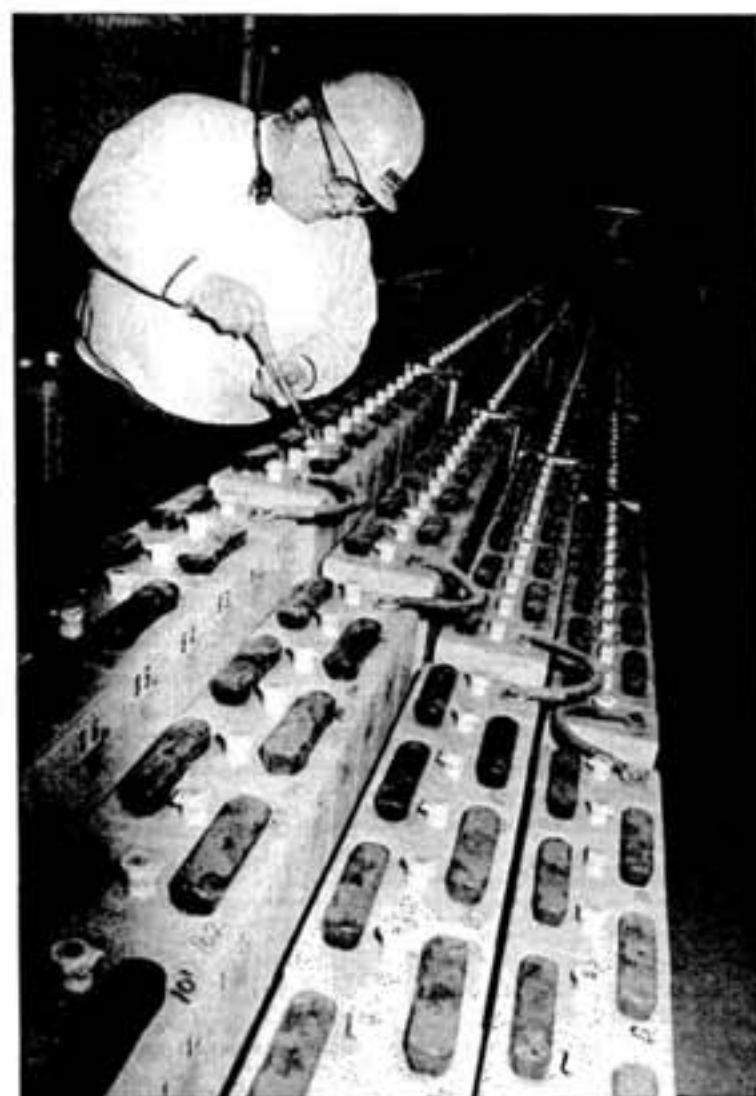
Ray Newman, maintenance electrician, checks the acid content of batteries in the Motor Generating Building of the Copper Cliff Smelter. Sixty-year-old motors were removed and replaced with 730 nickel-cadmium batteries. In the case of a power failure, the batteries supply power to six converters, which turn molten metal in the smelting process. The previous back-up power system for the converters was a seven-ton flywheel, which would continue to run for about 20 minutes in a power outage.
