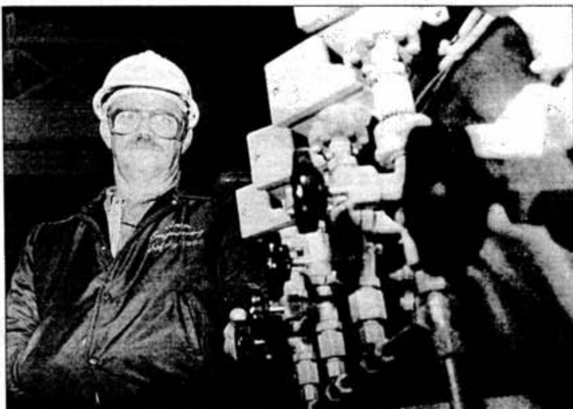
Ron Capstick, conversion project coordinator at the Smelter, likens the Voith controller at No. 1 Powerhouse to an automatic transmission system for the air blowers at the Smelter. The blowers can now be turned on and off when needed thanks to the new 60 Hz power system.
