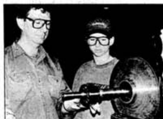
Machinist Terry Sasseville of Divisional Shops shows son Kyle, 14, how to install a new bearing on a water pump assembly.
