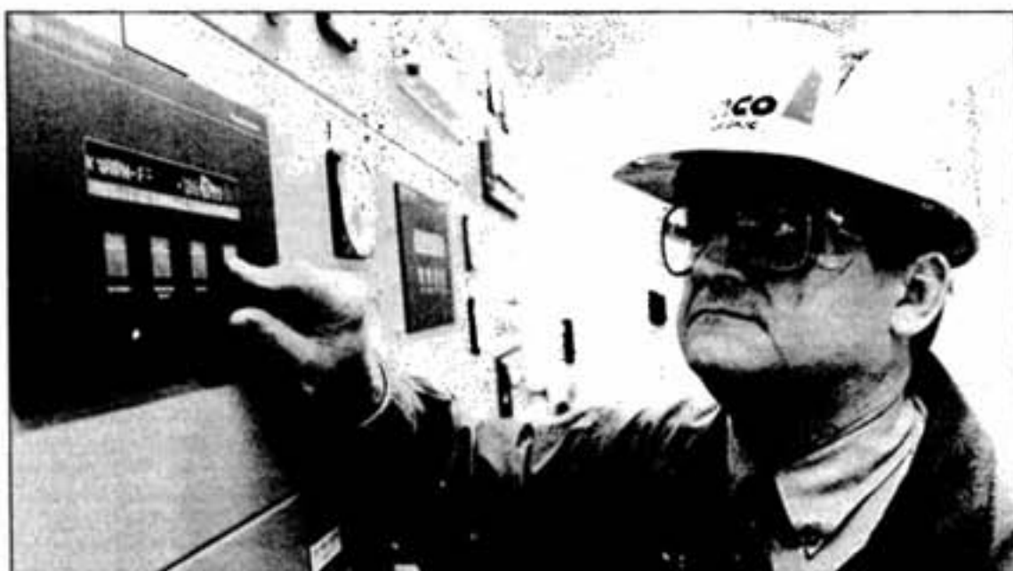
Stan Zajc checks conditions on the control wall inside the High Falls No. 1 power plant, constructed near the turn of the century and recently converted from 25 Hz to 60 Hz generation.
