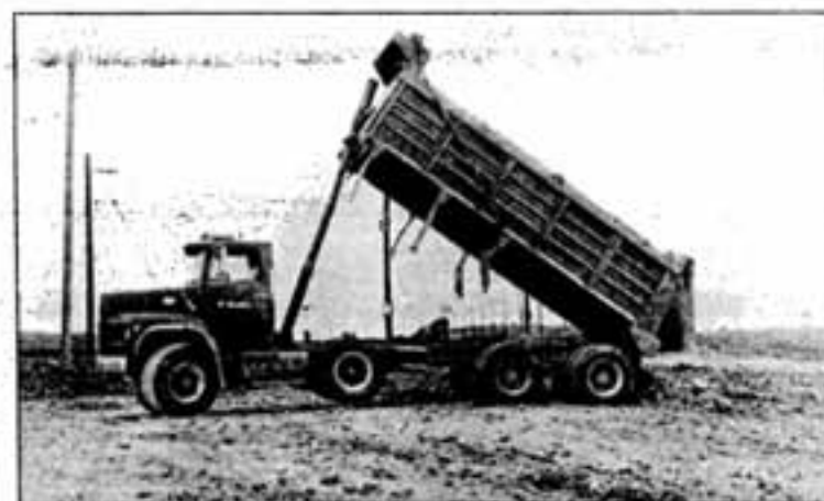
Before the slope could be seeded, trucks and graders were busy capping the area with 21,000 cubic yards of clay.
