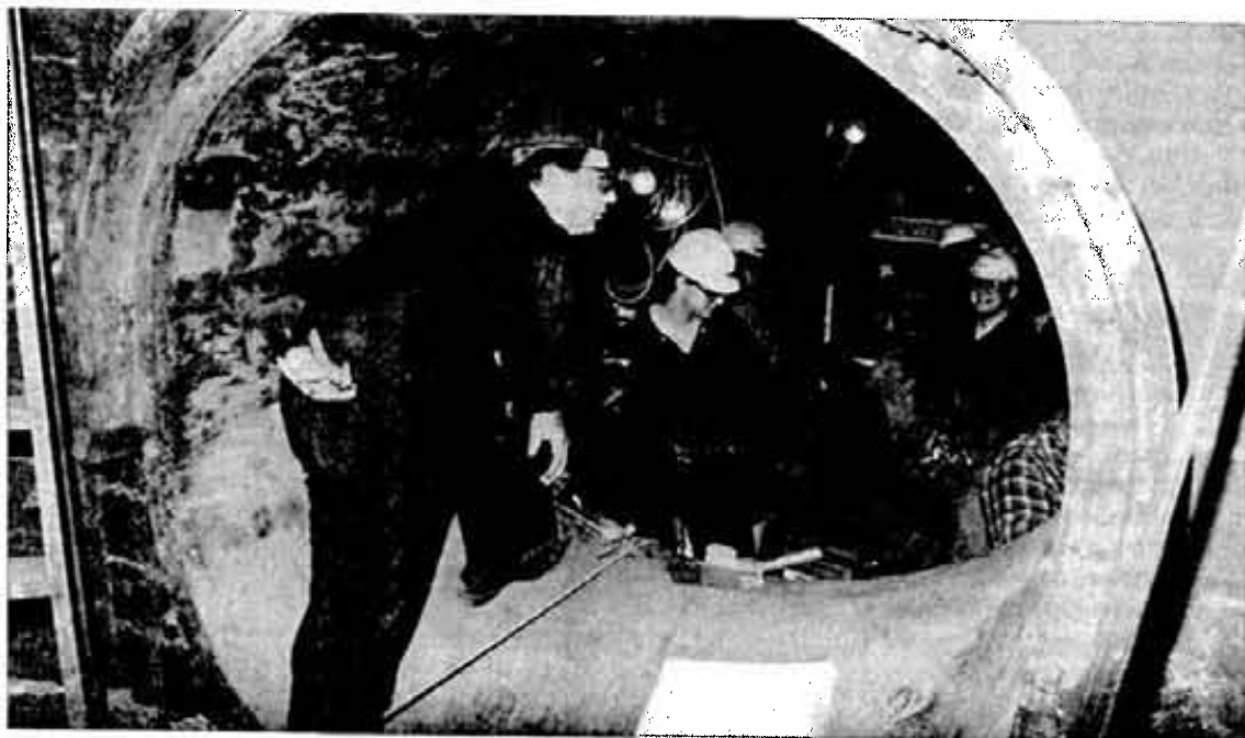
Malcolm Leger, process laborer, looks over the work of contractors who replaced brick and were adding ram lining to insulate No. 2 Flash Furnace. During regular operation, the furnace must withstand heat of more than 2,200°F. The maintenance work provided a rare view inside the furnace at the Copper Cliff Smelter.
