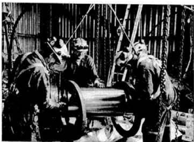
Working on a headsheave replacement job at Crean Hill Mine, are, from left, industrial mechanic Alvin Punkkinen, welder Patrick Thaxter, industrial mechanic Tim Weatherley and maintenance foreman Ellwood Hamel.
