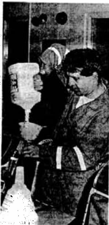
Peter Buratti fills his BG 174 breathing apparatus with soda lime during the bench test portion of the competition.
