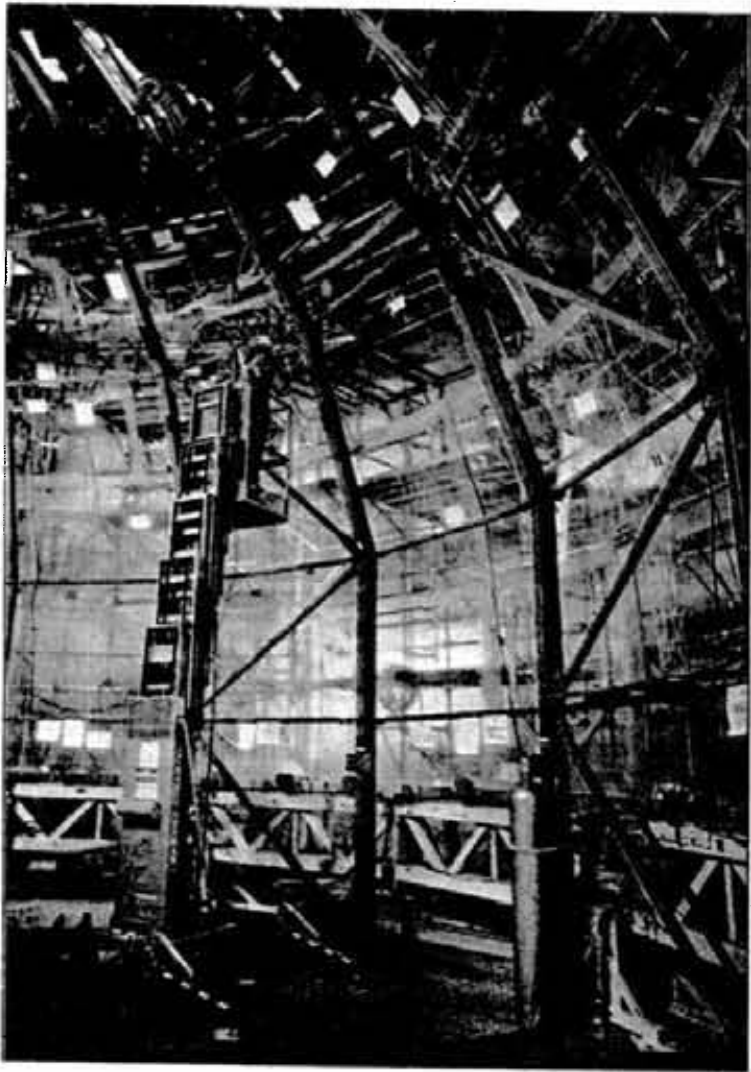
Mark Tokarsky of the Sudbury Neutrino Observatory polishes the acrylic vessel in anticipation of the ceremony marking the completion of the vessel's upper hemisphere.
