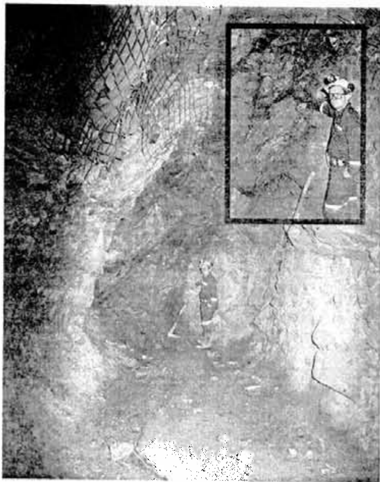
Looking like a mini-version of Inco's bulk mining drifts, this small drift is a good example of narrow vein mining. Inset shows McCreedy chief mine geologist Chris Davis beside the vein running vertically to the left of his hand.
