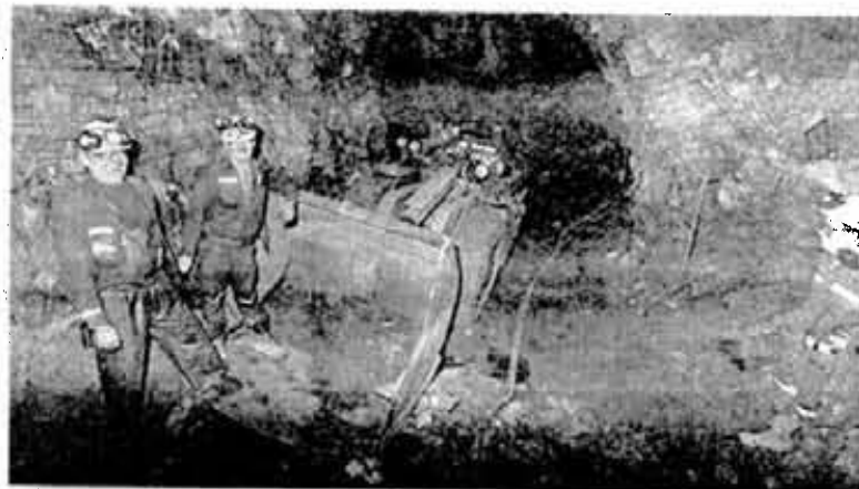
Development miners Charlie Annett and Ron Hanlon stand in the bucket of a two-yard scooptram that looks like a toy compared to Inco's huge scoops used for bulk mining.
