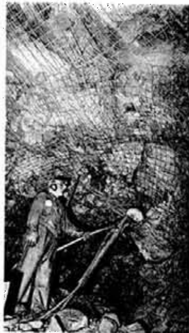
Development miner Charlie Annett bolts and screens a narrow vein heading. The vein can be seen clearly over his head.
