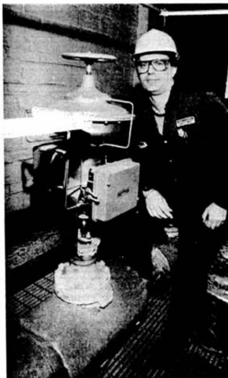
Alf Doherty stands behind one of the pressure control valves that regulate the amount of steam going through the pipes.
