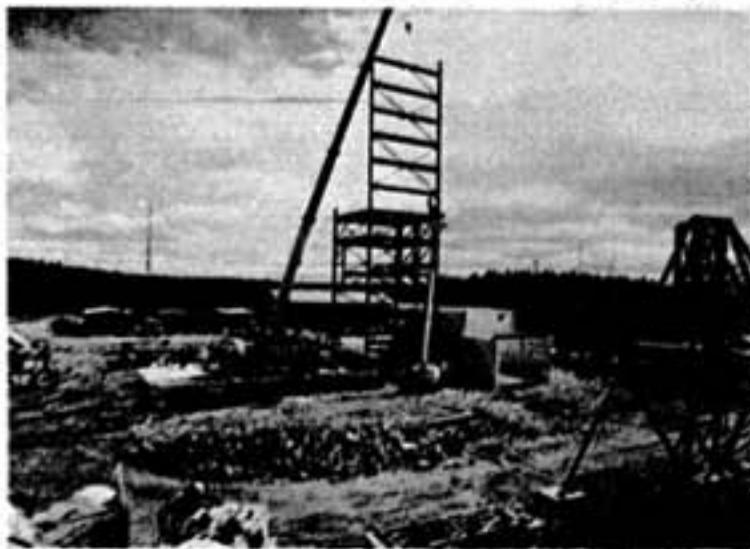
Taken from approximately the same spot, these views show the transformation of the Victor site. At the top is the clearing of the ground. The centre picture shows the installation of the shaft collar form (circular drum-shaped object centre left). The final view shows the erection of the headframe.
