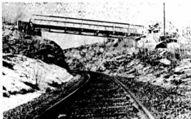
A Bailey bridge replaces a timber bridge over CNR lines. The bridge serves as a road that Inco uses to transport equipment and materials to the Victor site.
