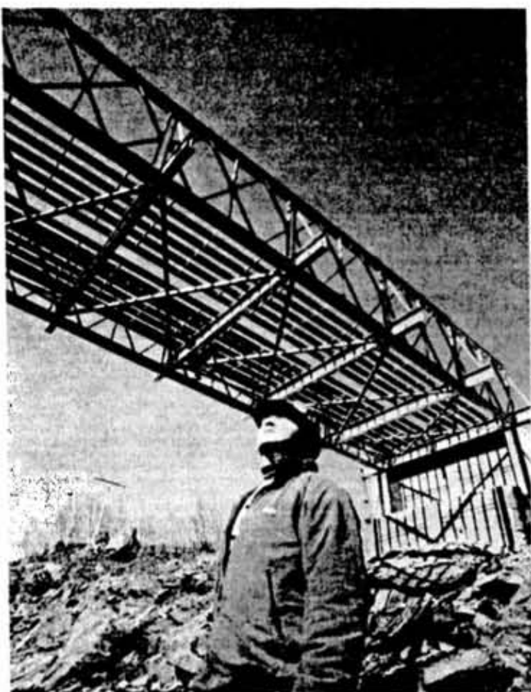
Victor project manager Bill Dawson stands under a new Bailey bridge that took a crane less than 20 minutes to lower in place but took months of preparation, scheduling and planning.
