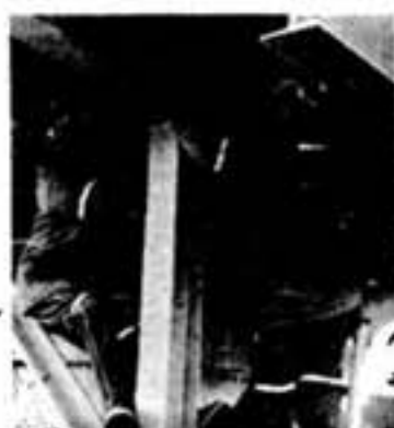
Welder Wayne Mohammed, left, and industrial mechanic Pat Matthews bolt the bottom beam of the heater house to its steel support structure.
