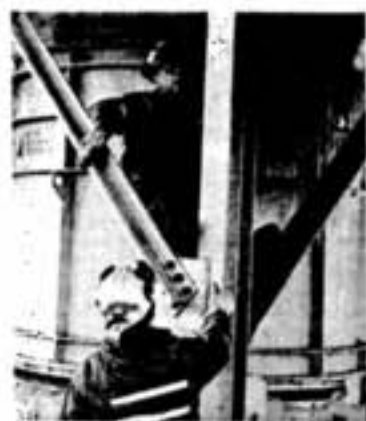
Pat Matthews gets up for a closer look as he guides the heater house into proper position for final tie-in to the permanent steel supports.
