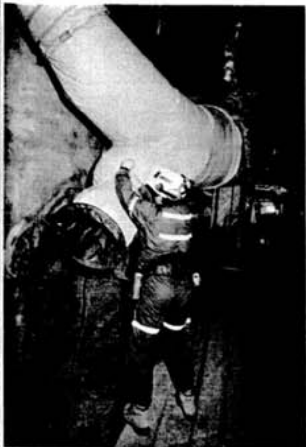
A workman installs a ventilation pipe that brings cool air to the people working in the huge cavern. At 6,800 feet underground, the temperature can get as high as 90 degrees fahrenheit.
