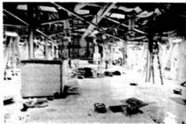
This structure, at the top of the cavern, provides access to the huge acrylic vessel that will hold 1,000 tonnes of heavy water.
