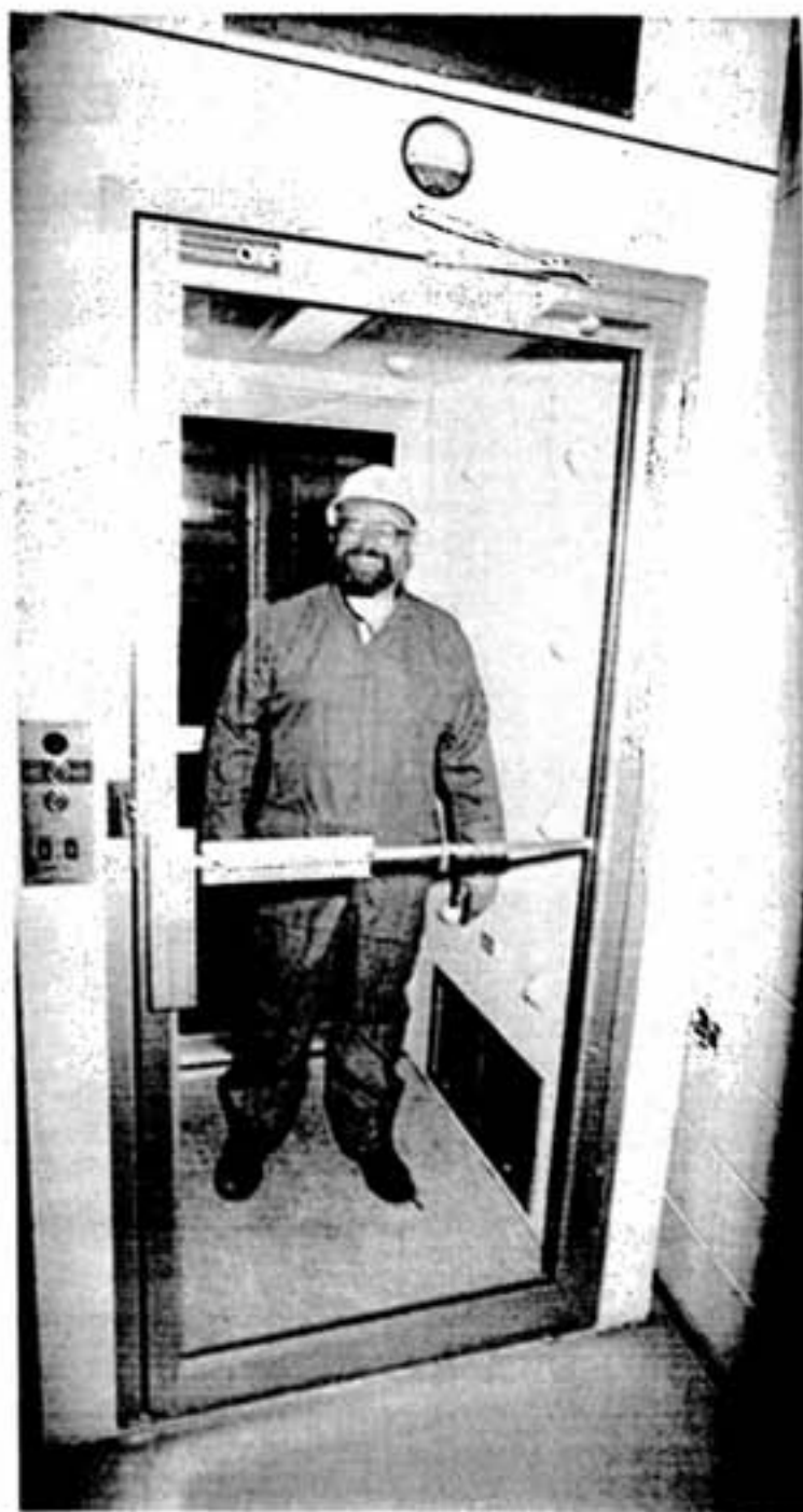
Who turned off Dave Schroeder's water? Nobody. This is an air shower that blows any remaining dust off the specially-designed anti-lint and anti-static coveralls.
