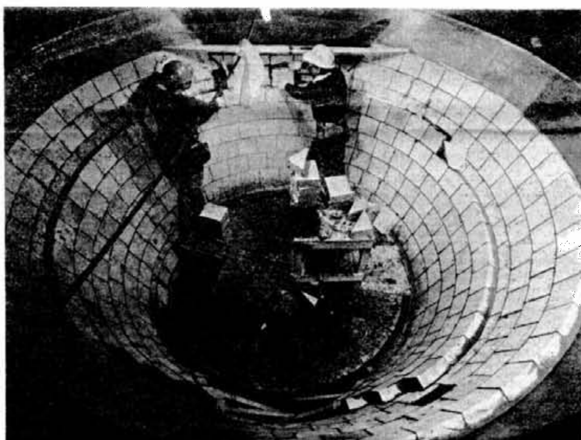
Workmen lay brick inside the quench chamber for No. 2 Flash Furnace, part of Inco's $600 million Sulphur Dioxide Abatement Project which applies the latest technology to meet Inco's environmental goals. Environmental, safety and production enhancements have changed the face of Canadian mining.
