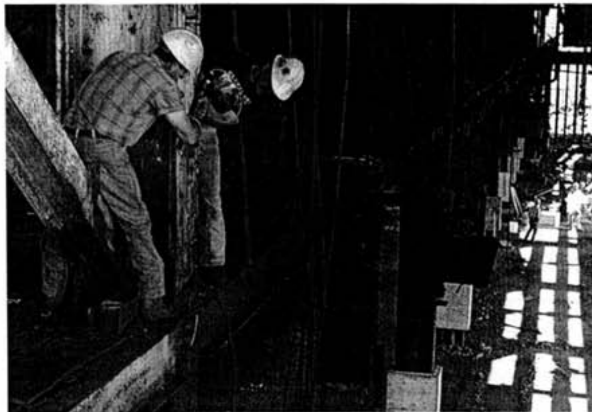
Explosives are attached to girders above building ground floor.
