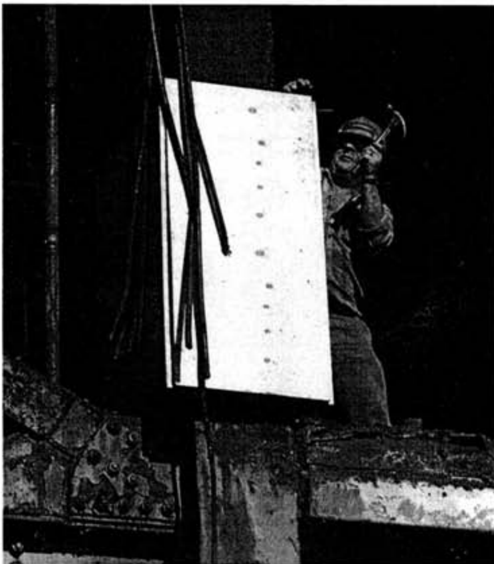
The explosive charges are protected from premature detonation by adjacent explosions with a wood box.
