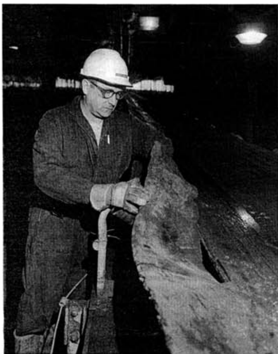
Clarabelle Mill laborer Ray Leblanc shows what a piece of tramp steel in the muck can do to a conveyor belt.
