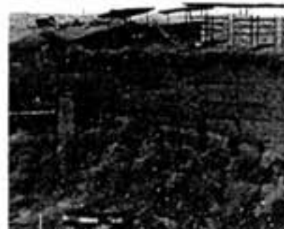
The initial explosion (note flashes on lower left of structure) sets off a timed series of charges encased in wood boxes attached to girders along the bottom of the structure.
