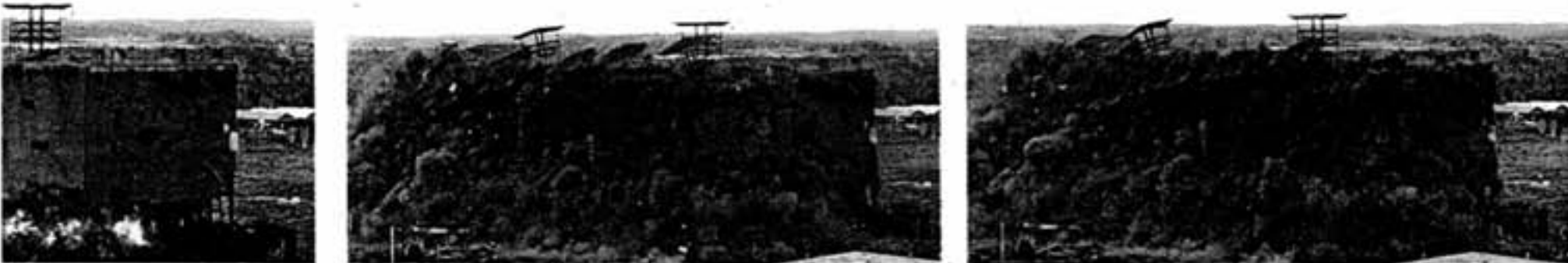
tom of the building. The boxes prevent the explosives from being detonated prematurely by adjacent blasts that "walked" in timed sequence
