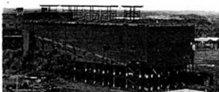
The initial explosion (note flashes on lower left of structure) sets off a timed series of charges encased in wood boxes attached to girders along the bottom of the structure.
