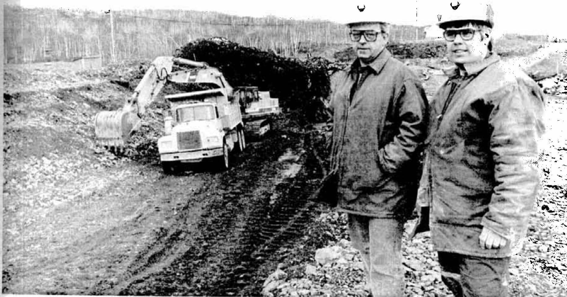
Andy Noel and Cecil Munroe at the site of the last berm under construction. The earth had to be removed 34 feet down to bedrock, then clay added to form the berm.
