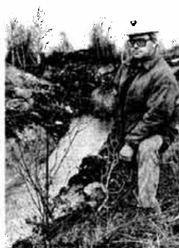
Andy Noel stands near one of the water diversion trenches dug to prevent water from seeping underground into Little Stobie Mine.
