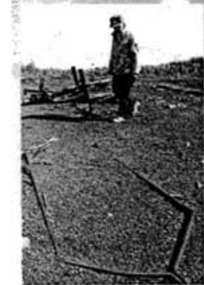
Marty Puro takes a closer look at a half-buried iron hanger used to transport tram cars along an overhead tramway. The car was suspended between the two open ends and the closed end hung on the overhead cable.
