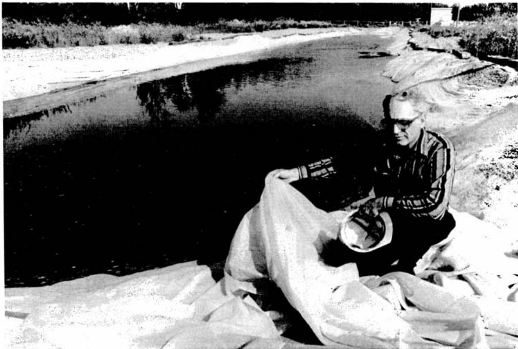
Fabrine lines the bottom of one of the recharge pits.
