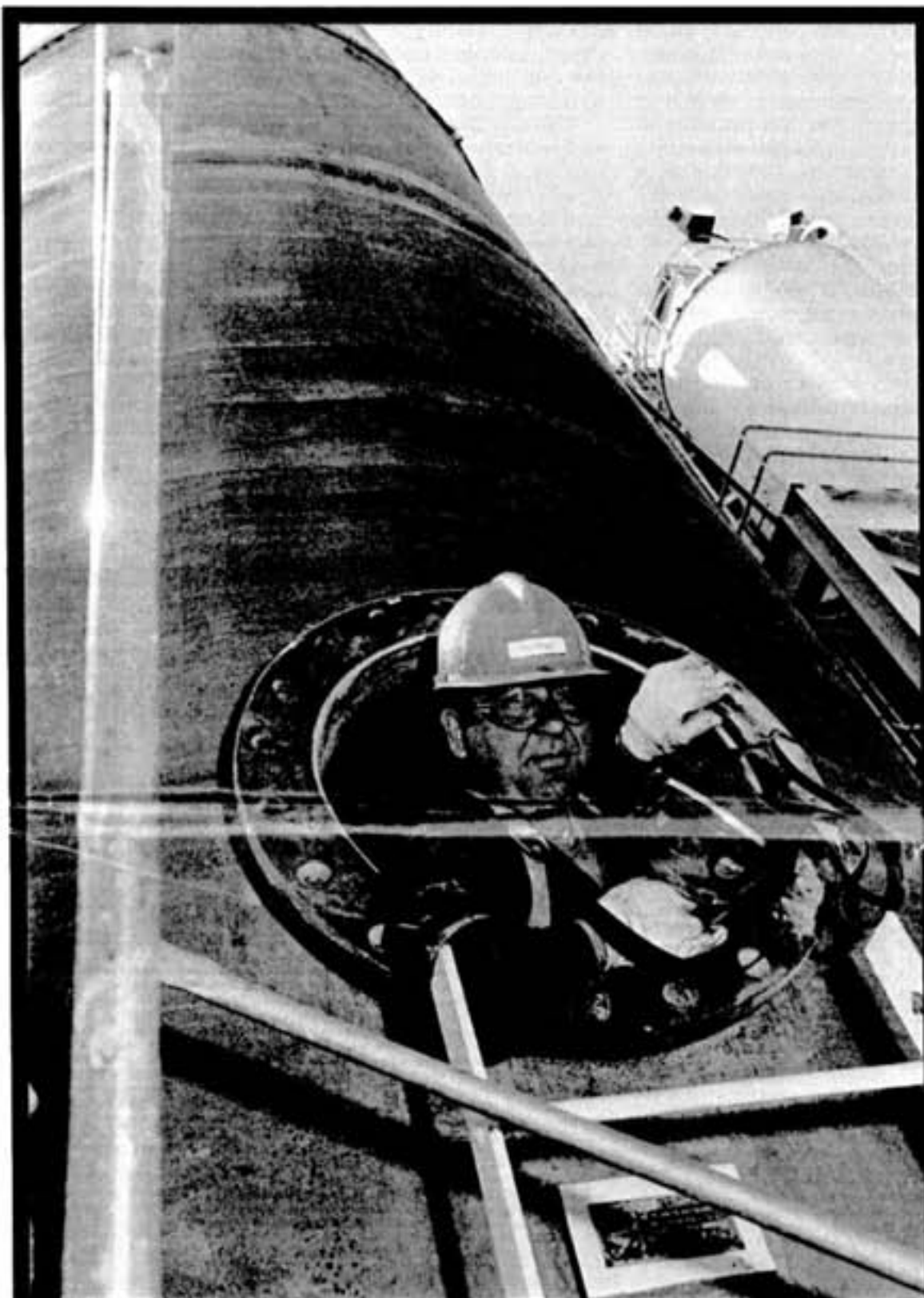
Maintenance mechanic Bob Airhardt emerges from the Port Colborne bulk storage tank after installing a heating coil used to dry copper/nickel silica oxide slurry before shipment to Sudbury. The new drying process replaces air-drying in an outside pond that took up to eight months. The new method takes a week, allowing the Port Colborne slurry truck to return to Copper Cliff fully loaded.
