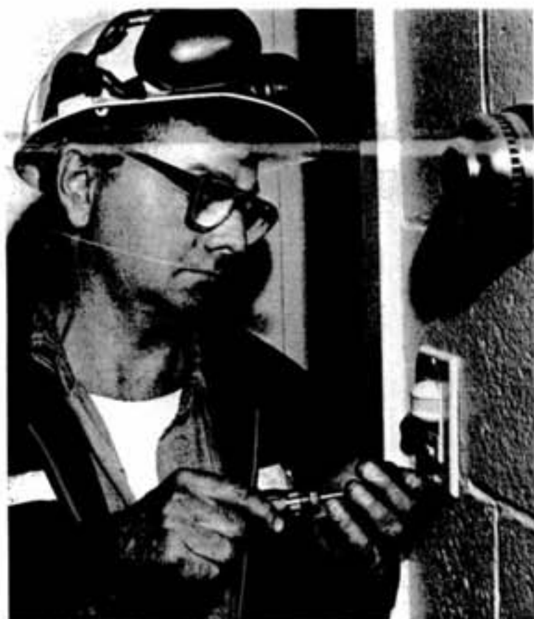
Electrician Gerry Willmott installs a motion sensor that triggers room lights.
