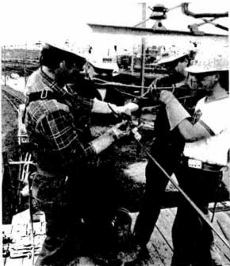
A Power Department crew replaces trolley wire on a section of rail near the Parker Gate from the top of a specially-rigged rail car. About 10 miles of the copper wire that carries voltage to power Inco's electric locomotives was replaced during the shutdown. From left, Fern Poltras, Lloyd Meadows, Gerry Courtemanche and Tom Eles.
