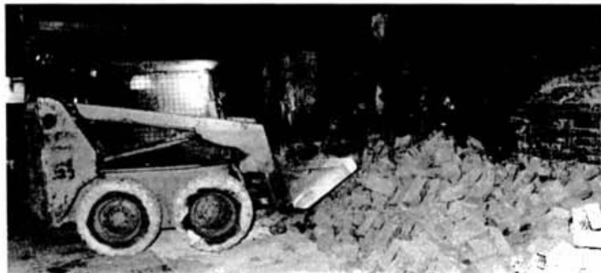
No. 6 reverberatory furnace side wall brick is removed during an annual furnace demolition shutdown project at the Smelter. The walls are rebuilt with new brick in time for the resumption of operations.
