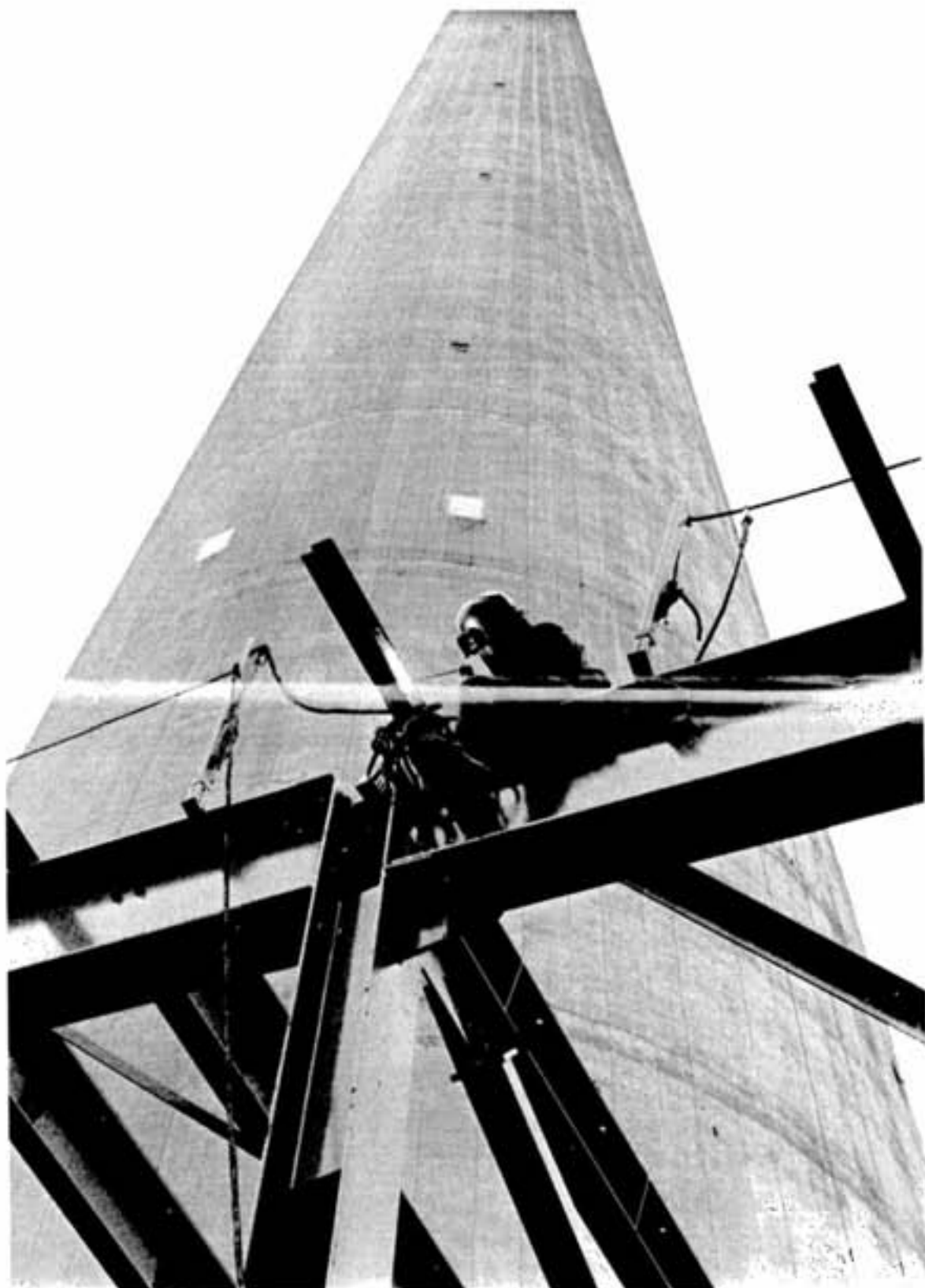
At the base of the Superstack, a welder runs another bead along a section of I-beam. The Sulphur Dioxide Abatement Project again made the Smelter the busiest place in the Division during the shutdown.
