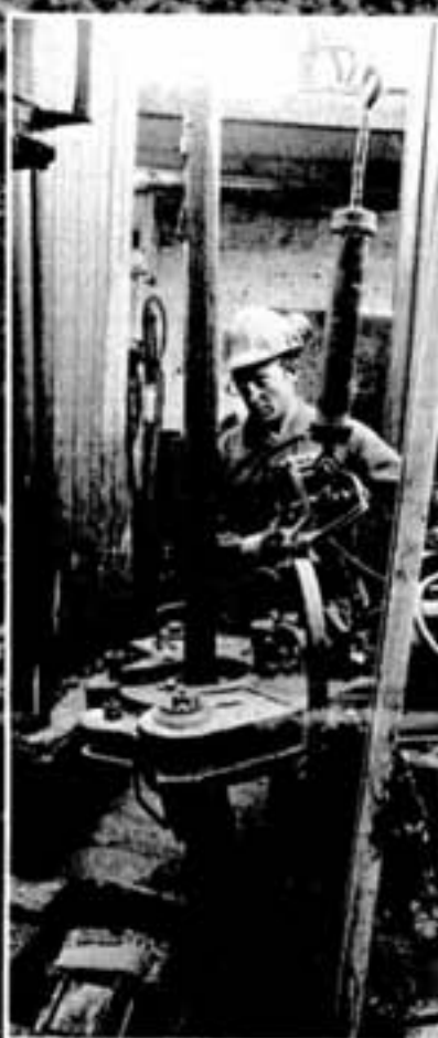
Driller Richard Despatie with tubings logs used to 'break' rods as they come to the surface. This one comes from 6,510 feet below the surface.
