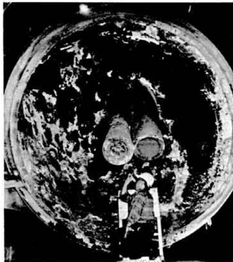
Foreman Don Martin checks nickel refinery hood flue.
