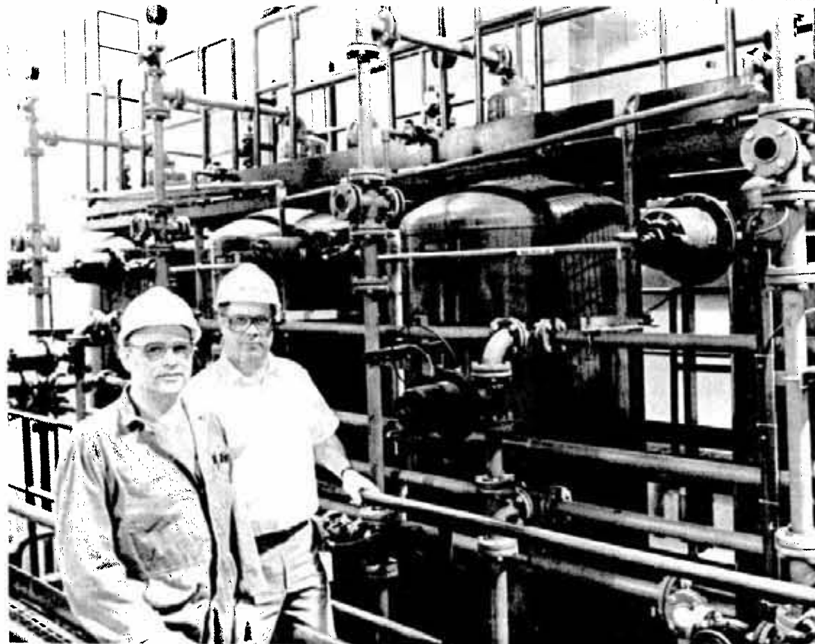
Port's Italo Rossi and Mark Pataran at the mixing columns where nickel is extracted.
