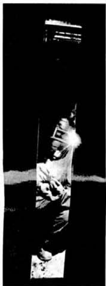
Welder Donald Hache welds steel for the tap hole on a new Copper Refinery furnace.
