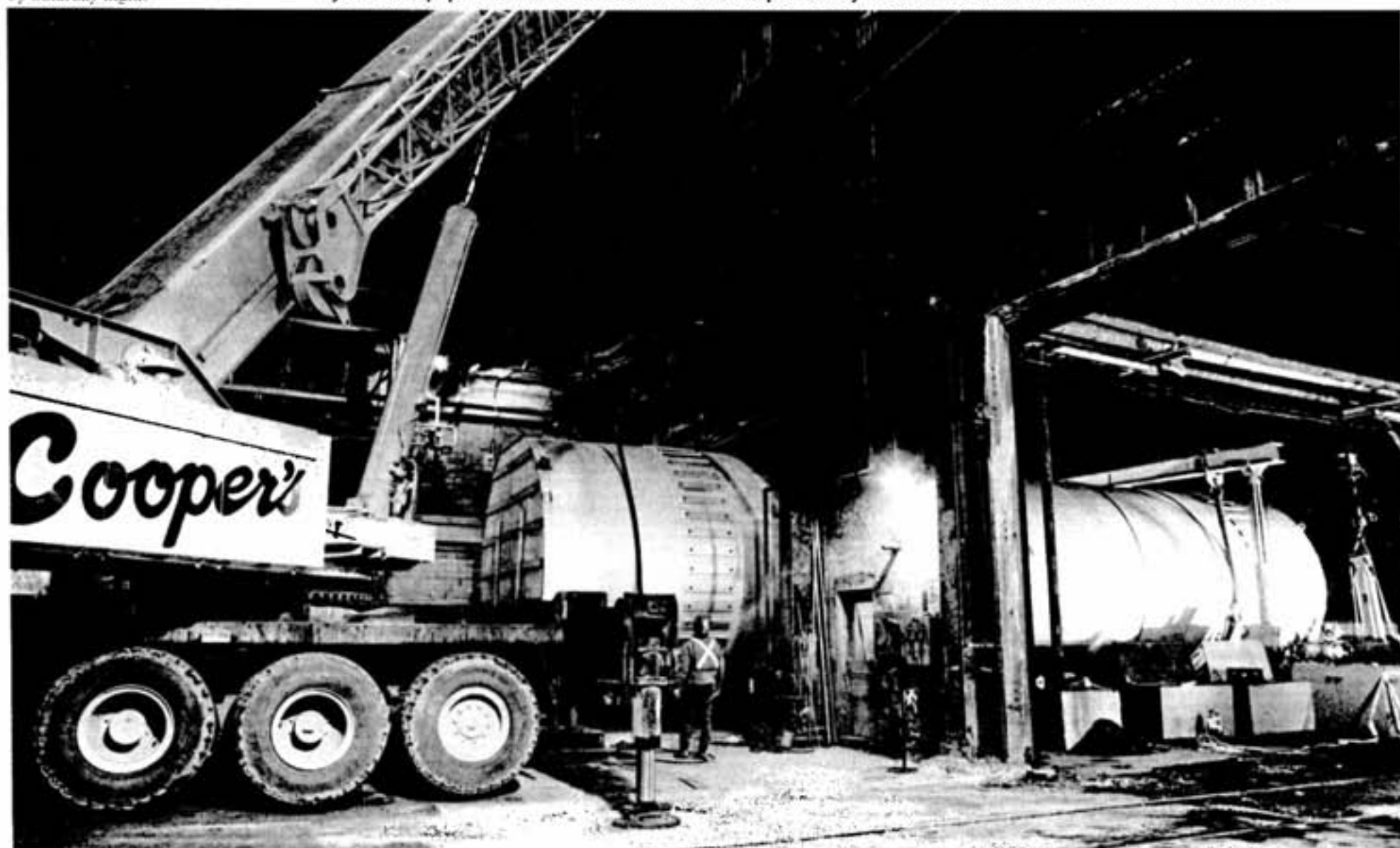
Hydraulic equipment moved the melter shell onto previously installed concrete cradles on the Smelter floor.
