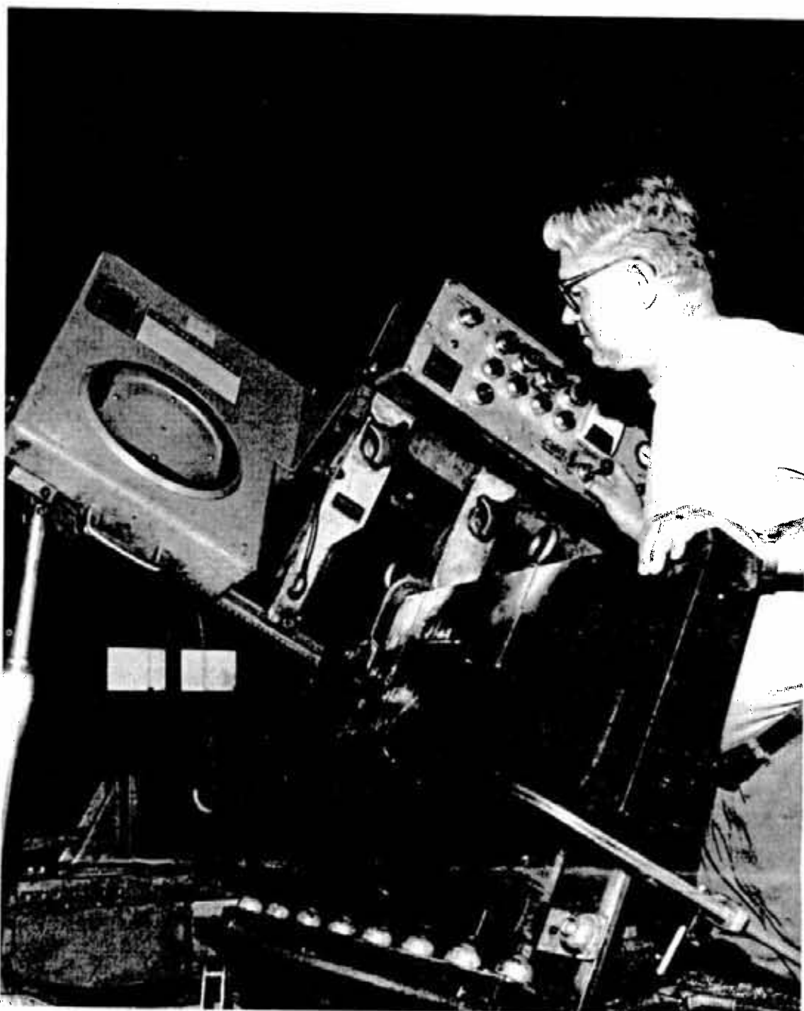
Machine operator Marcel Dupuis cuts an expansion joint with a horizontal saw.
