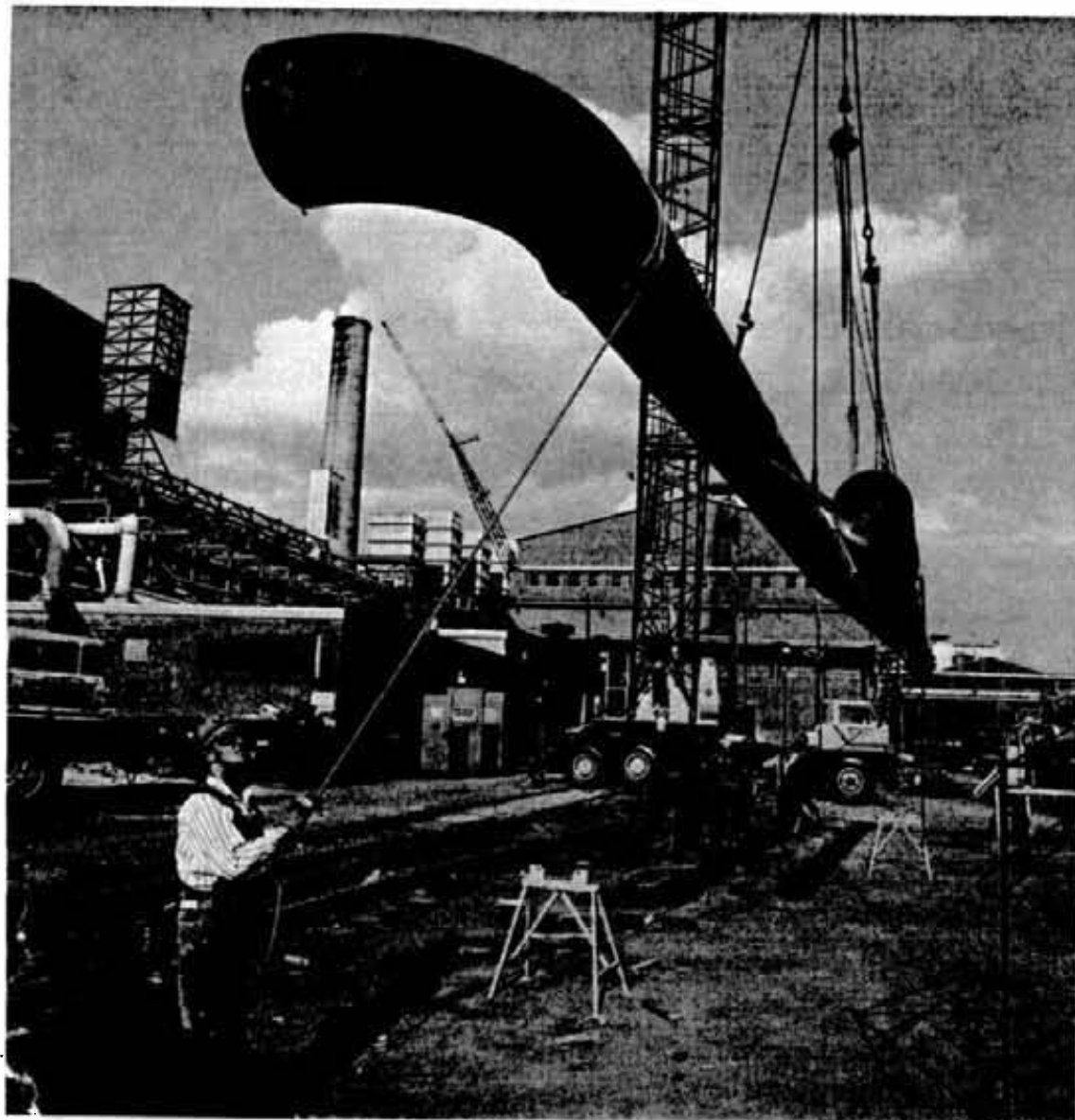
A huge oxygen pipe is maneuvered into place for installation at the smelter.
