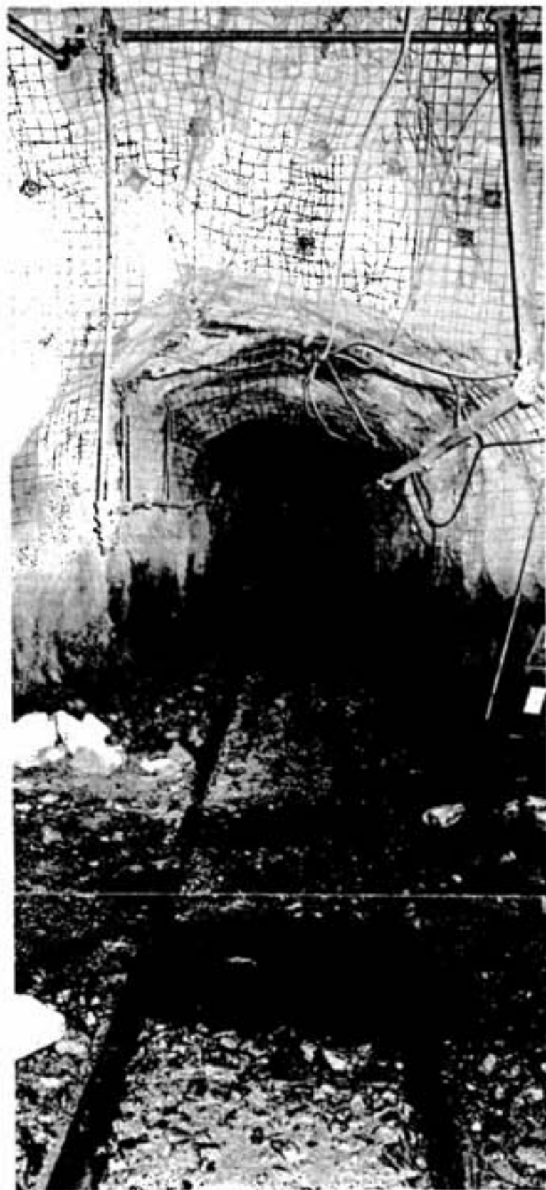
The old Little Stobie drift is dwarfed by new opening (foreground) to make room for the huge electric automatic haulage truck (right, top opposite page).
