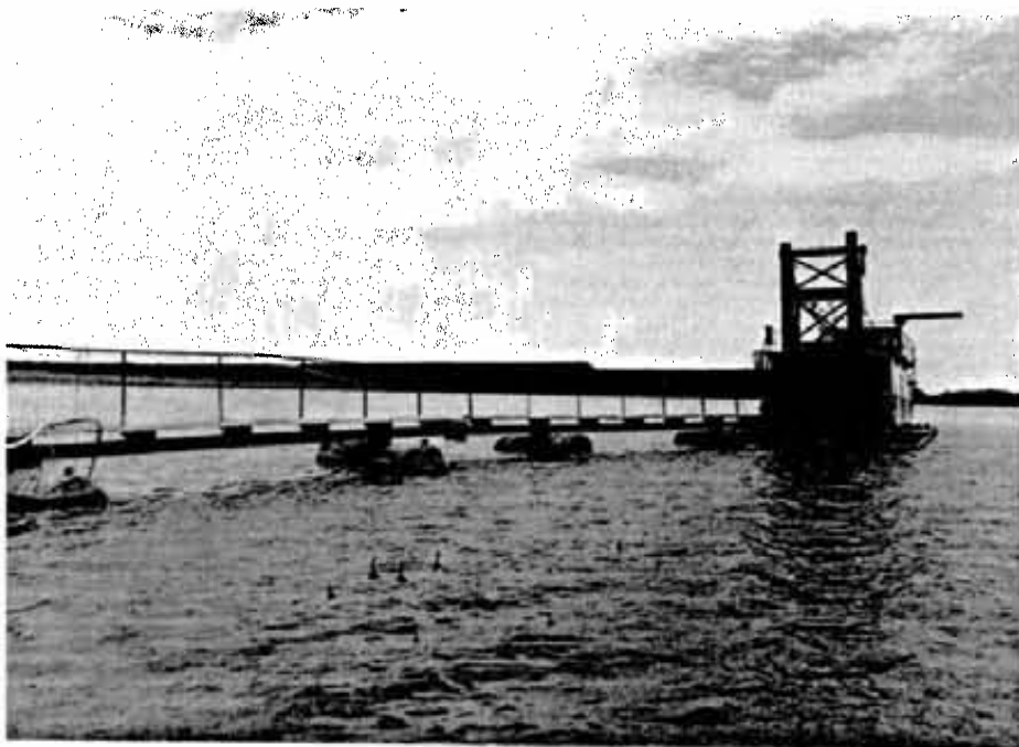
Pipeline from dredge feeds silt to shore.
