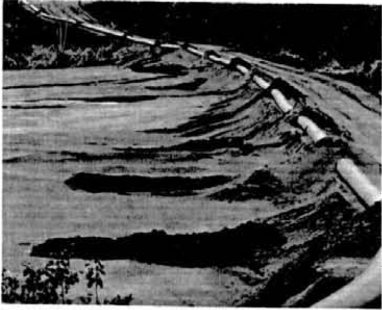
Miles of pipe transport tailings to site
