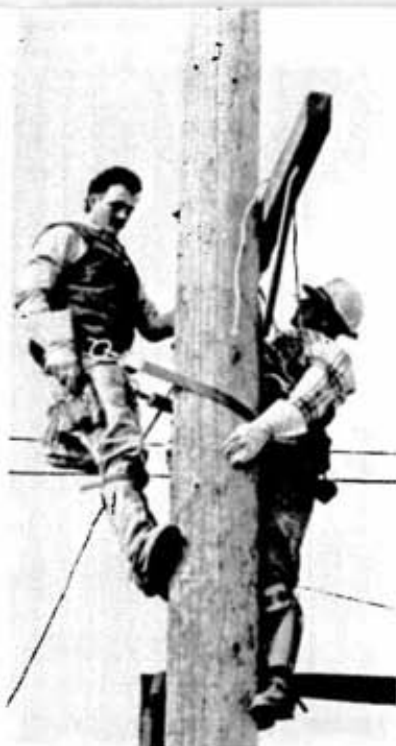
— The proper way to rescue an injured line-man was demonstrated
