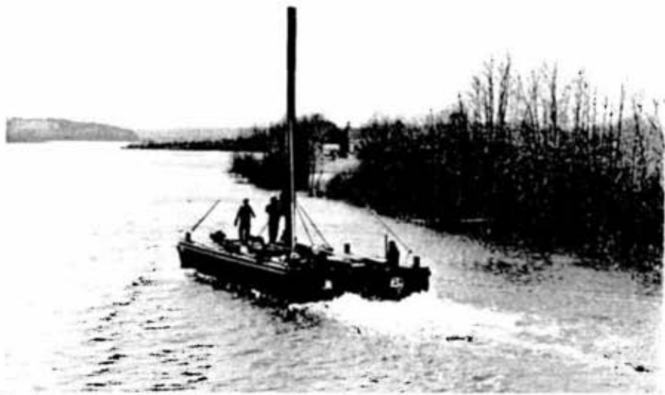
The barge, with a temporary hydro pole in place, was moved into place and sunk.
