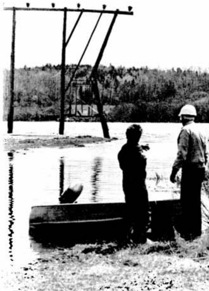
Jack Hunter and Laurent Rancourt inspect the damage inflicted on a hydro pole by a huge ice flow on the Vermillion River. All three poles of another set were completely demolished.
