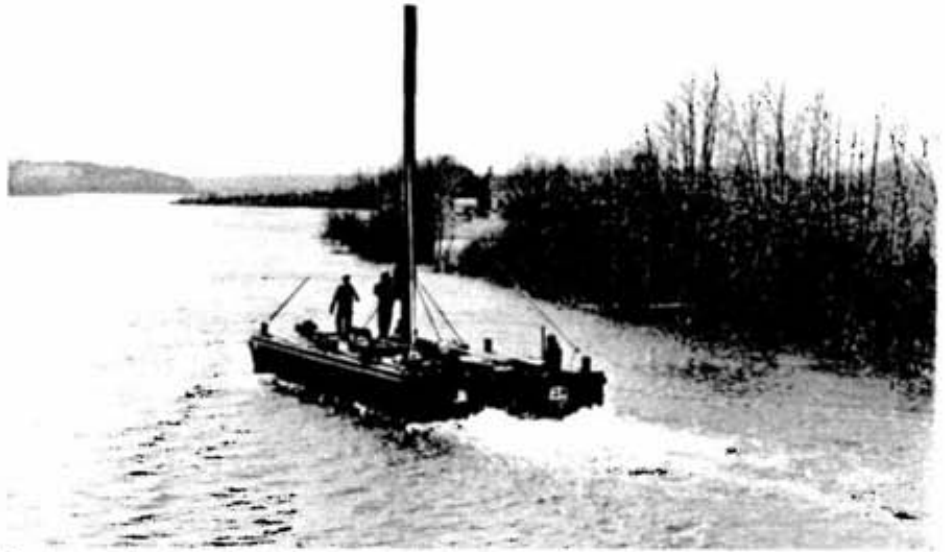
The barge, with a temporary hydro pole in place, was moved into place and sunk.
