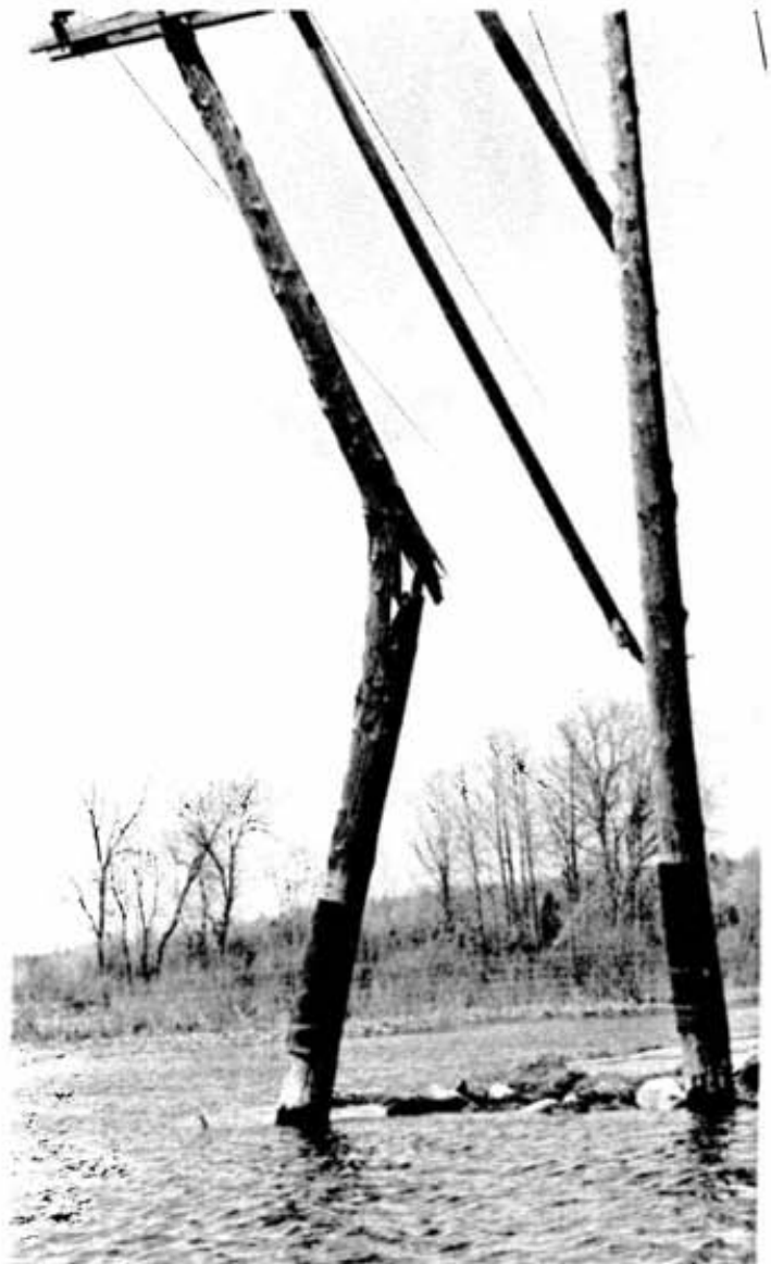
A closeup view of the snapped hydro pole.
