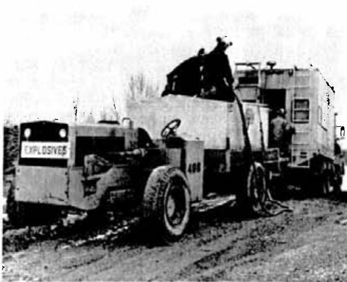
Tim Dupuis, mechanized stope driller, and Lawrence Caverly, construction leader, fill a hopper on the back of a scissor lift truck with the pumpable emulsion manufactured in a mobile plant. Gilbert Prieur, assistant plant operator for Ireco checks the progress at the mixing truck.
