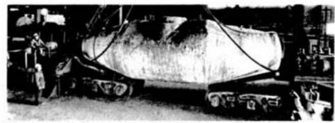
Slings are maneuveured into position by craneman George Viaux in order to lift the hot metal car off its base.
