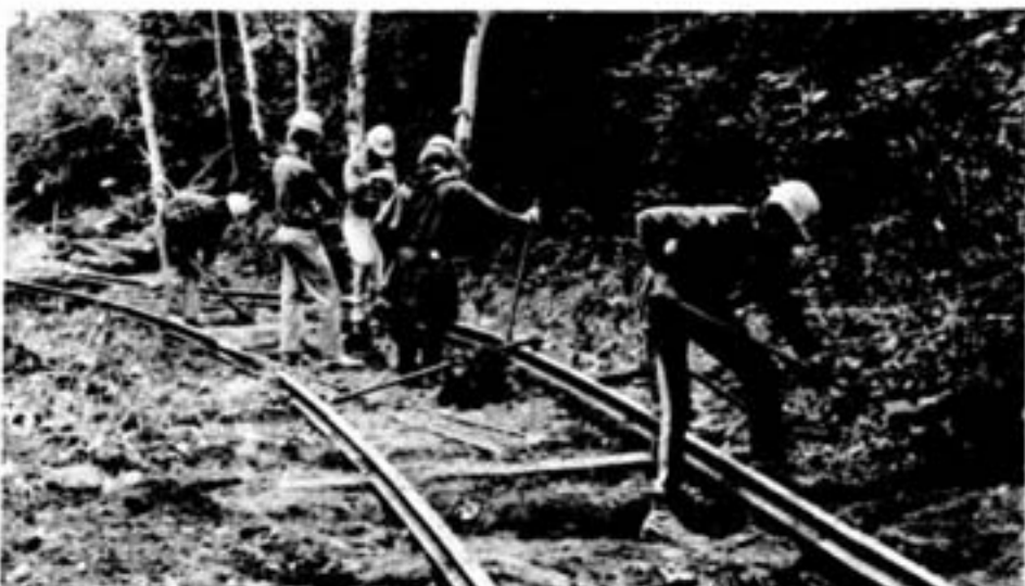
Part of the rehabilitation of the marine railway by this crew of junior forest rangers involved replacing old, worn railroad ties with new ones.
