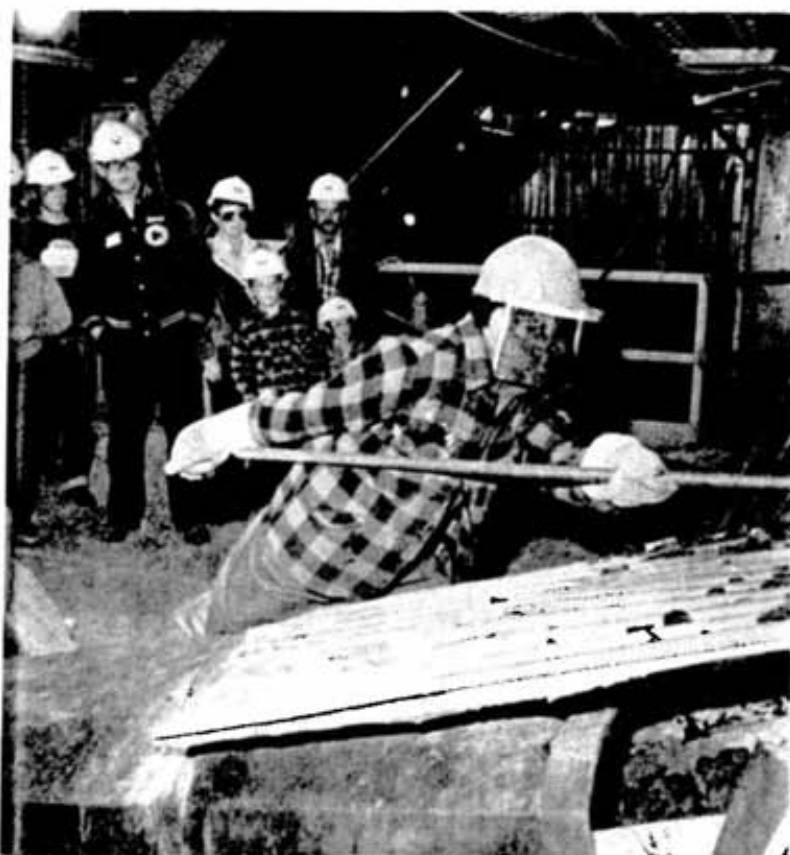
A group of young visitors watch a skimmer do his work on the skimming platform of a furnace as Scott McDonald explains the process.
