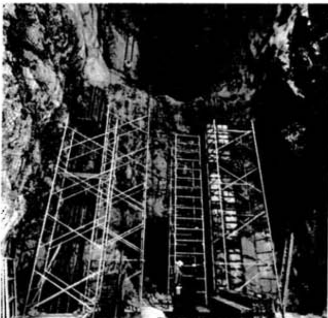
Four crusher floor supporting columns in an early stage of construction.
