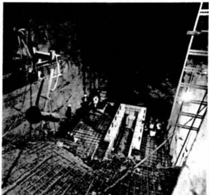
Pipe is prepared to pour concrete for the crusher floor.
