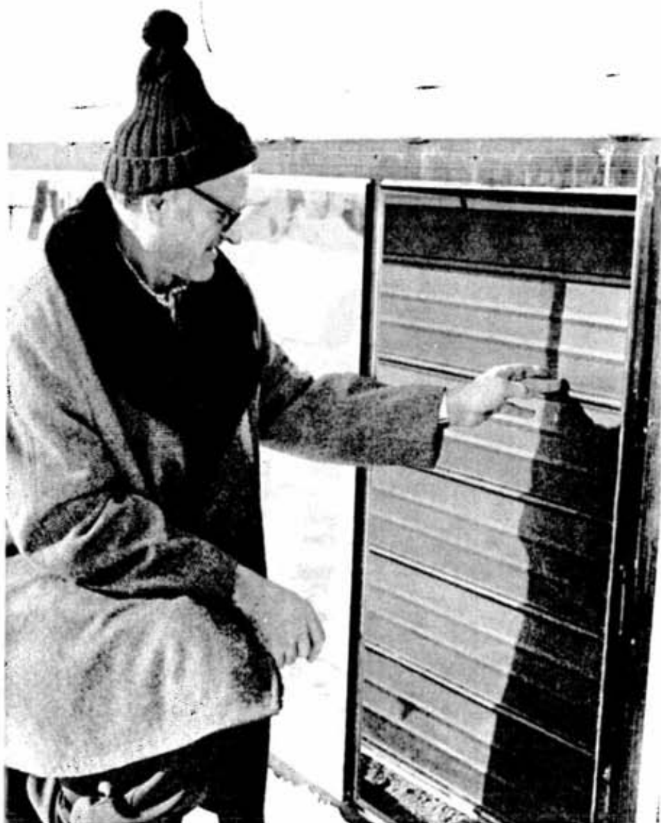
Ed shows how the duct connects to the fan which forces warm air from the panels into his house.
