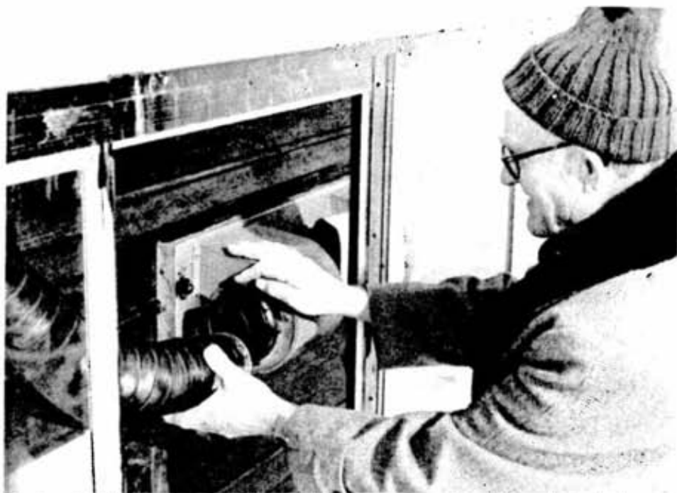
Ed shows how the duct connects to the fan which forces warm air from the panels into his house.
