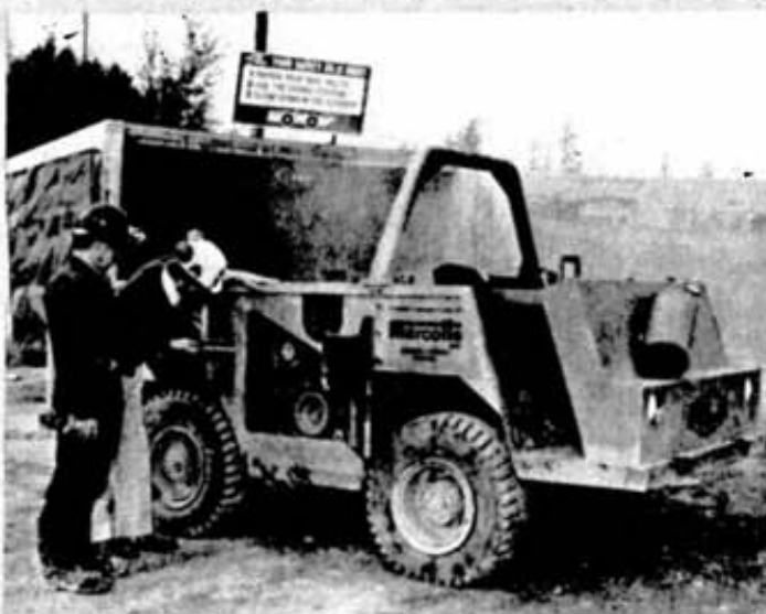
Ray Marcotte , left, of Marcotte Mining Machinery in Sudbury, and Gary Moore , superintendent of McCreedy west mine inspect a personnel carrier known as the Ram Car that was designed and built by Mr. Marcotte's firm.
