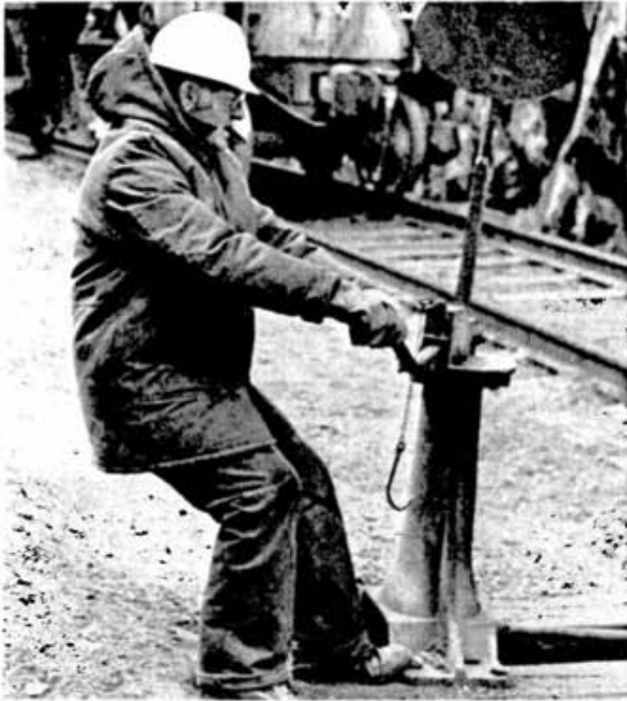
Eugene lines the track switch that allows the train access to the appropriate track. The switch target tells the engineer which way the conductor has lined the switch. Ray will move the loco only after he has received the proper signal to do so from his partner. The empty pots are pushed along the track that leads under the skimming platforms of the furnaces. A cable car puller system operated by smelter employees is used to "spot" the pots for loading.
