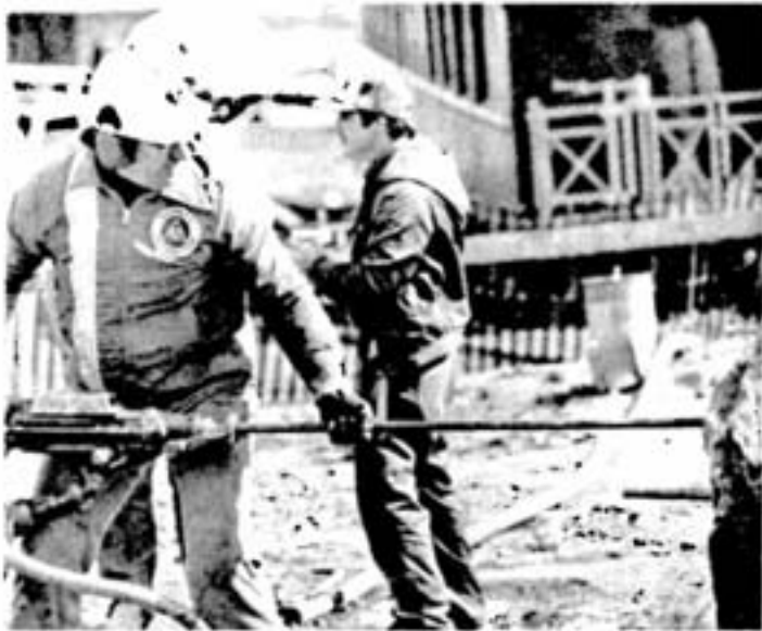
Racing against the clock, Inco's Marcel Henry aims the jack leg drill into the rock face.
