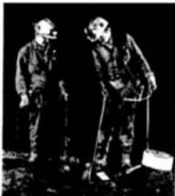
Loading a vertical retreat blast... Claude Courchesne, left, blaster boss, holds onto the wooden plug he will lower down the hole once Paul Henn, blaster helper, has completed measuring the hole.
