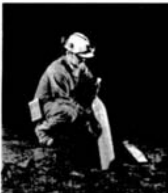
Claude Courchesne lowers the "sausage" of a blasting agent known as Aquamex into the drill hole.
