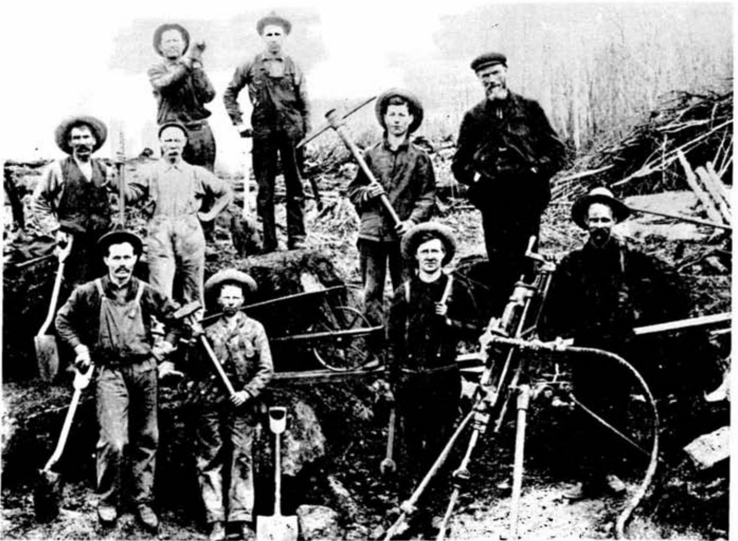
This was mining 1898-style. These employees of the Canadian Copper Company were surface mining an outcropping of ore near what today is Copper Cliff North mine. Picks, shovels and wheelbarrows were standard equipment as was the hand-cranked air-driven drill. Water for the drill was fetched by the pail.
