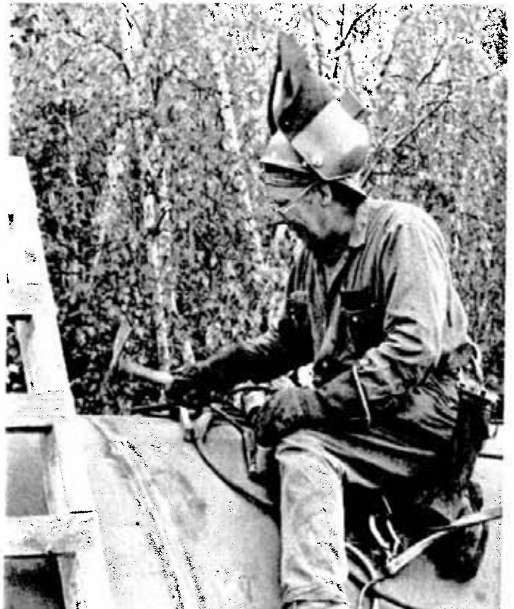
Specialist welder Vaino Ylitalo puts the finishing touches on sections of the penstock welded together.
