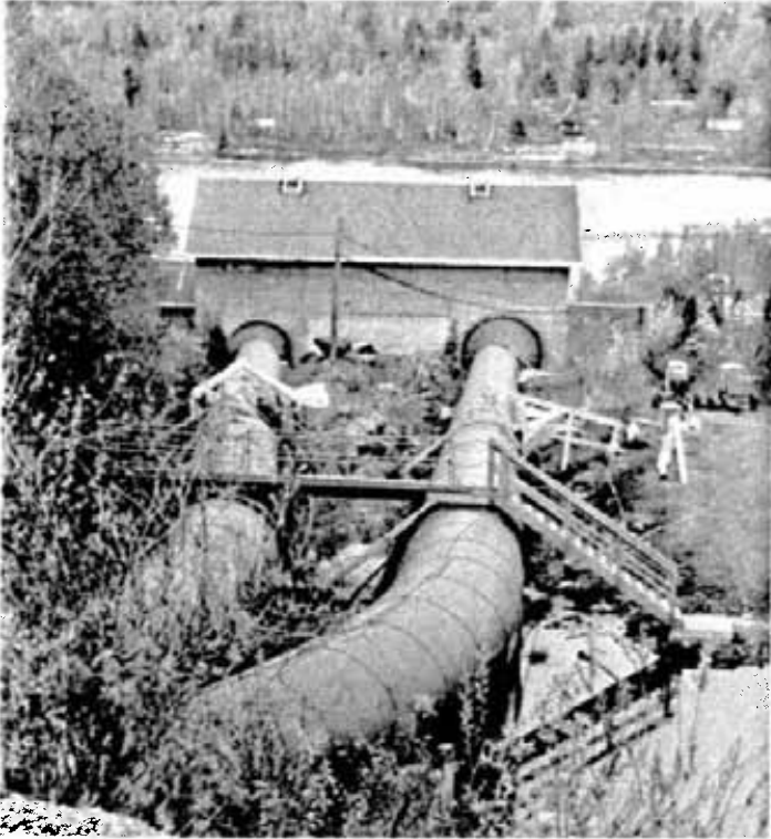
The penstock on the left required repair work after part of it collapsed. The building at lower centre is the generating station.
