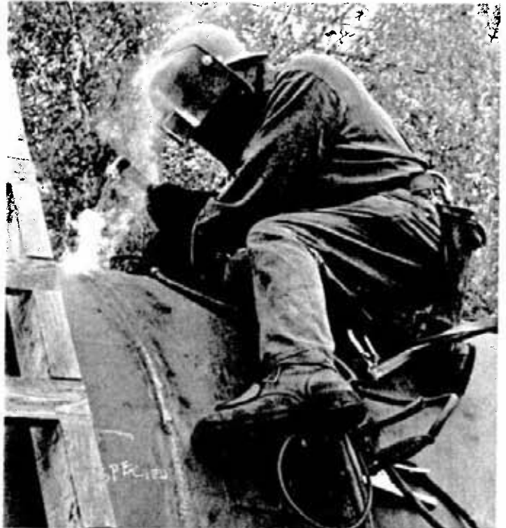
Specialist welder Vaino Ylitalo welds sections of the penstock together.
