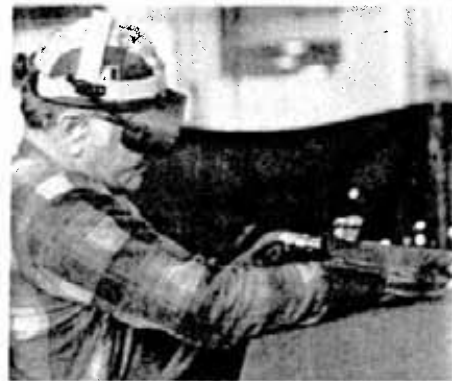
Cosimo Valenti, cuts a bolt off the converter collar during its construction at the plate shop.
