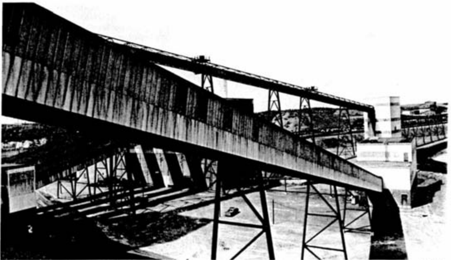
With the ventilation and heating revisions, ventilation air flows through the conveyor gallery from the mill tripper floor to the transfer house (right). From there, the air travels through the galleries to the crushing plant (left background), where it is directed to number nine hoistwell.
