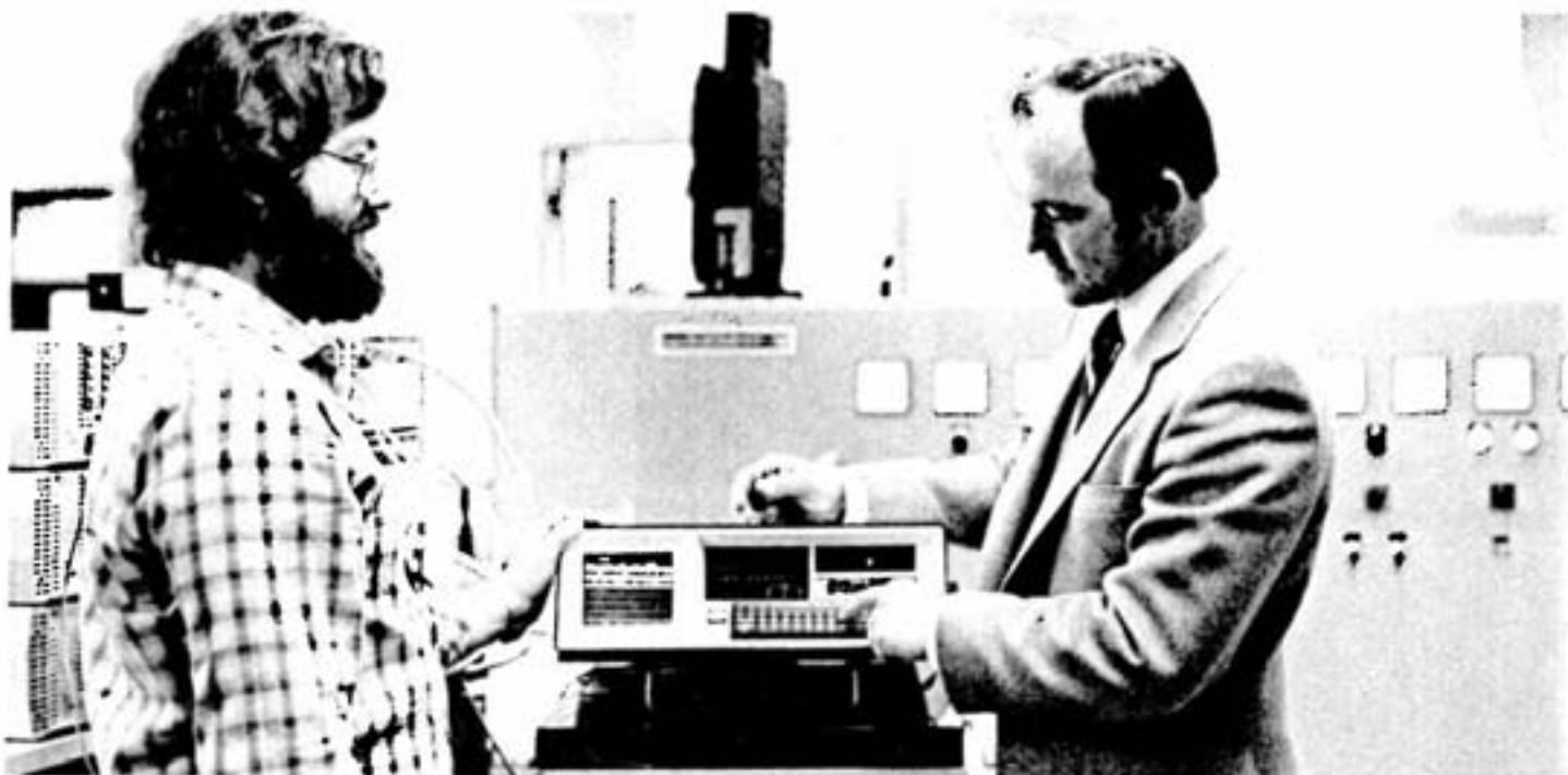
Computer services personnel Jim Giles, left, and Stewart Tait, operate diagnostic equipment used to test and monitor telephone lines between Copper Cliff and Thompson.
