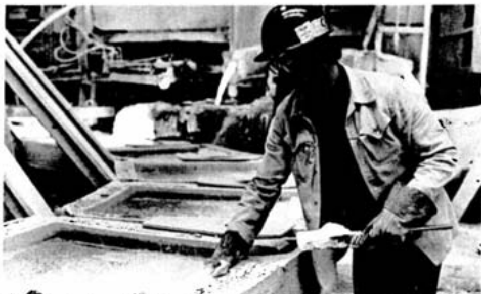
Suggestion plan winner Ray Morin applies powdered Barite 100 to the copper anode molds.
